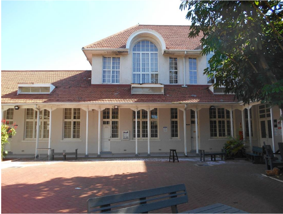
FIGURE 11: COURTYARD OF THE LISTED BUILDING
