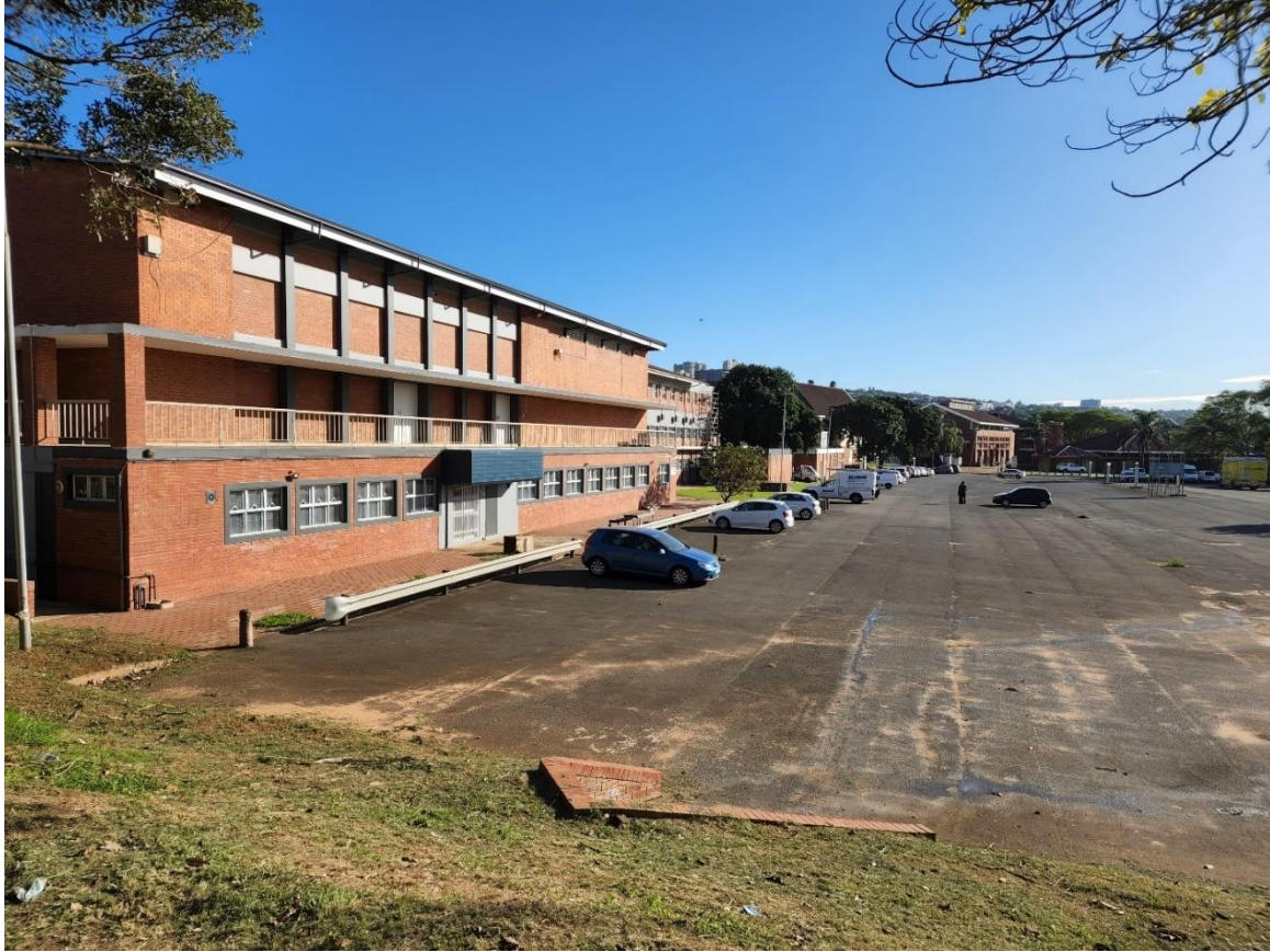
FIGURE 16: IMAGE SHOWING THE BACK OF MANSFIELD HALL
