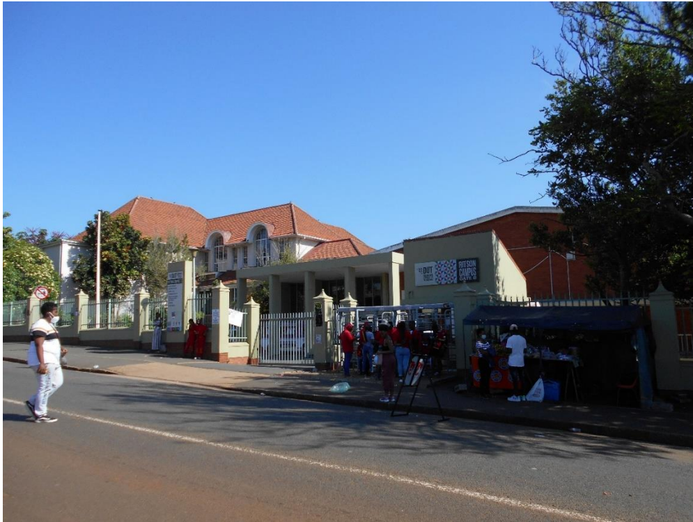
FIGURE 10: ROAD FRONTAGE OF THE LISTED BUILDING
