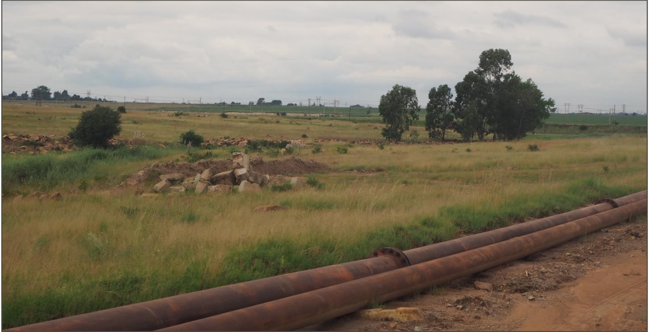
Figure 29 Pipeline on the Western Border of the Site
