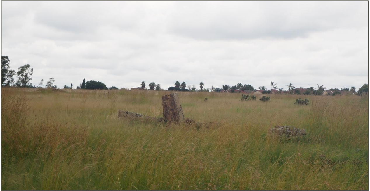
Figure 27 Dilapidated Mining Infrastructure
