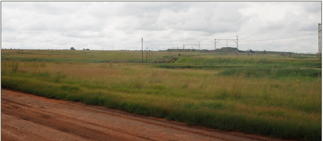
Figure 30 Railway Line on the Southern Border of the Site
