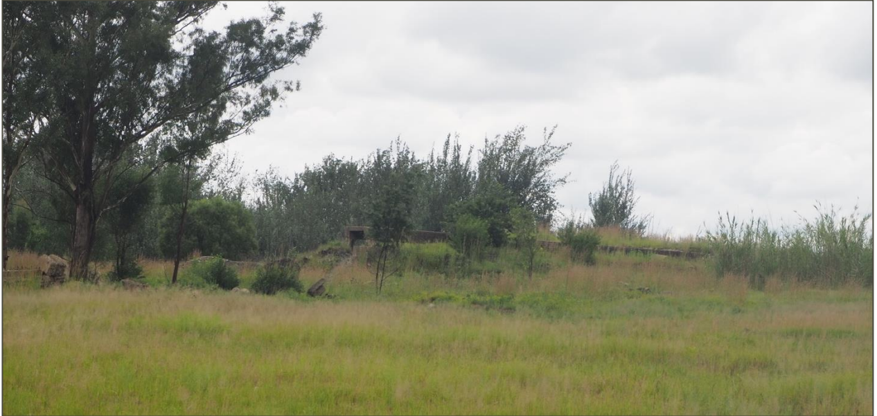
Figure 25 Dilapidated Mining Infrastructure
