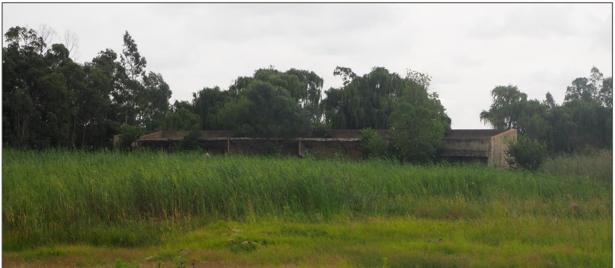
Figure 24 Dilapidated Mining Infrastructure
