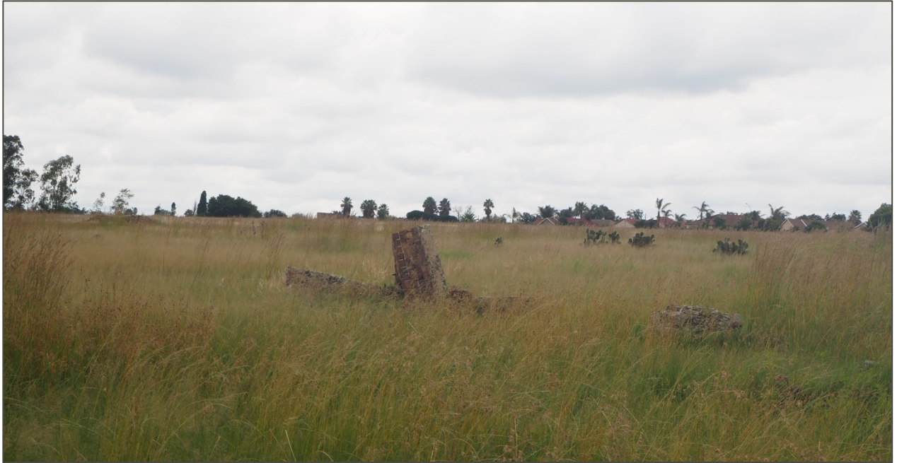
Figure 29. Dilapidated Mining Infrastructure
