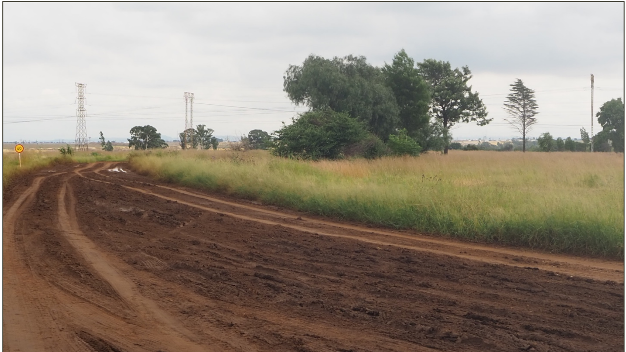
Figure 20. Access Road to Slimes Dam
