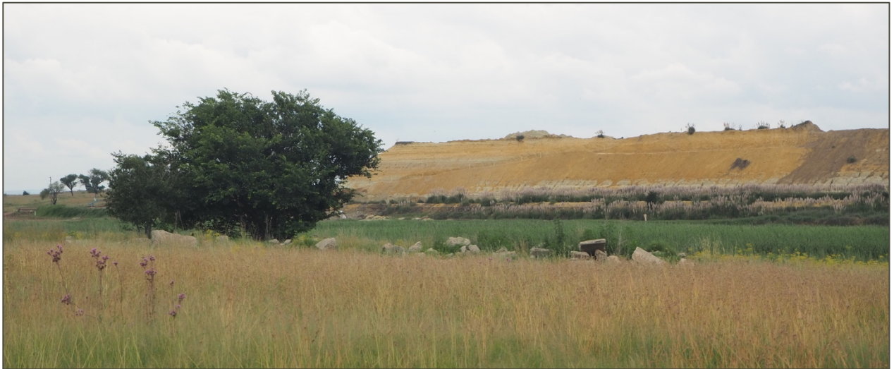
Figure 30. Slimes Dam on the Western Border of the Site
