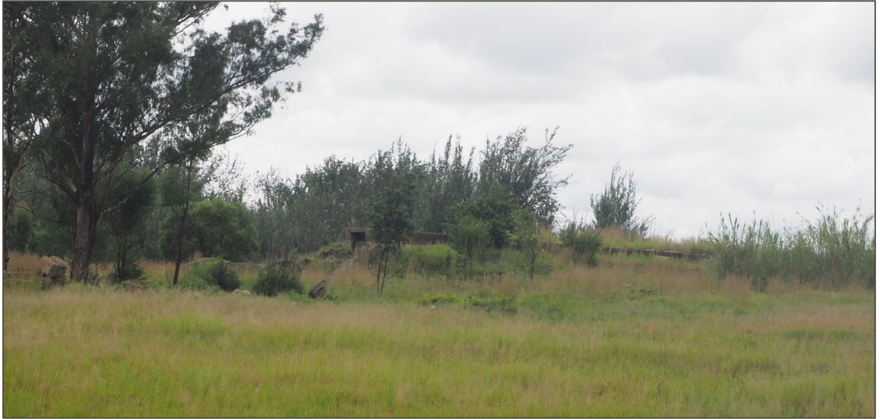
Figure 27. Dilapidated Mining Infrastructure
