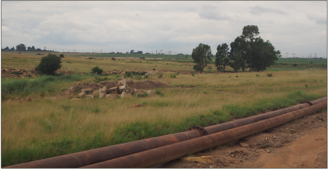
Figure 31. Pipeline on the Western Border of the Site
