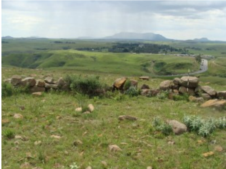
Figure 23: One section of walling on Site 9.
