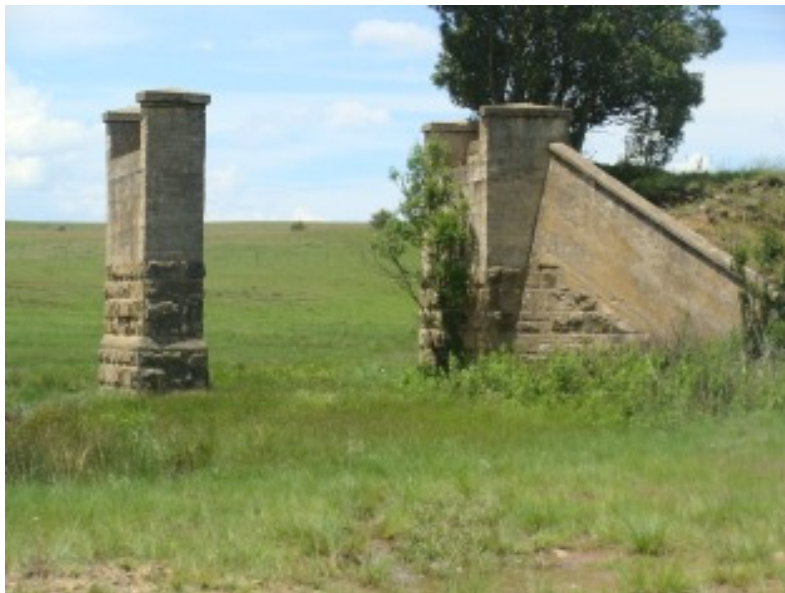
Figure 25: Closer view of bridge.
