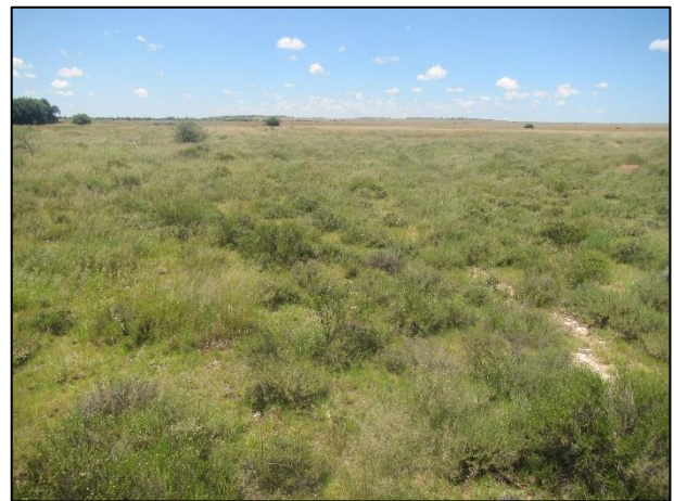
Figure 11: View east along the Braklaagte powerline connection.
