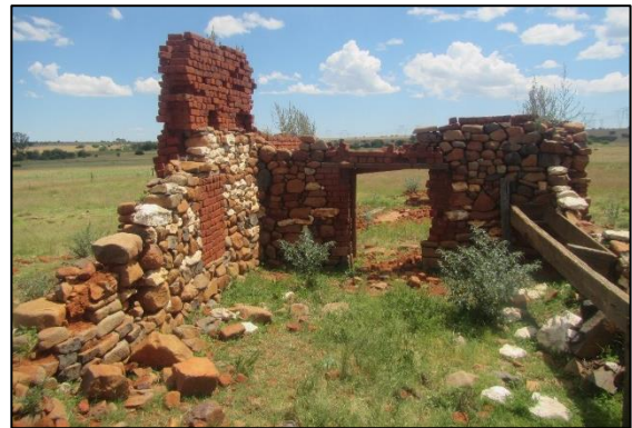
Figure 18: View of the smaller room of the ruined structure at waypoint 720.
