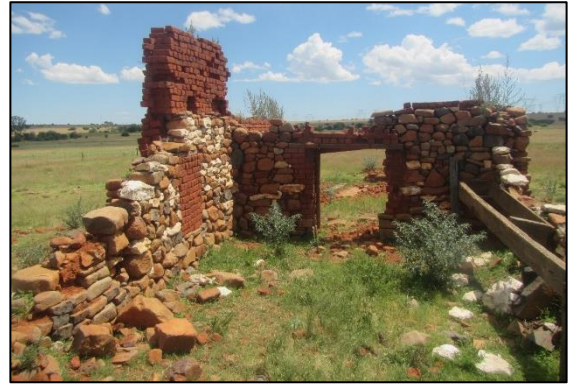
Figure 16: View of the smaller room of the ruined structure at waypoint 720.
