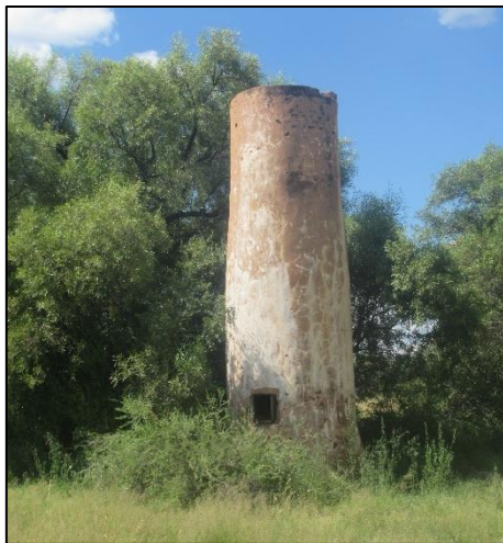
Figure 19: Ruined structure at waypoint 728.
