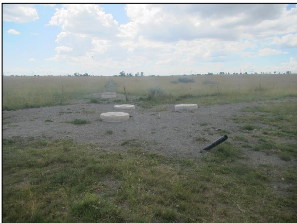
Figure 6: View northwest in Klipfontein 1 showing a buried pipeline route.
