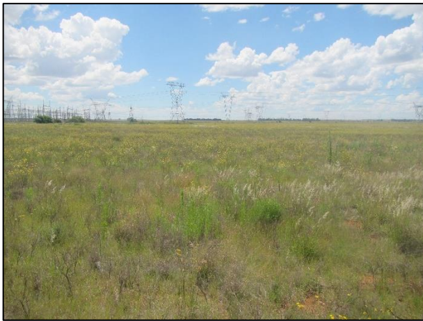
Figure 11: View north in the northern part of the powerline route with Perseus Substation visible in the background.
