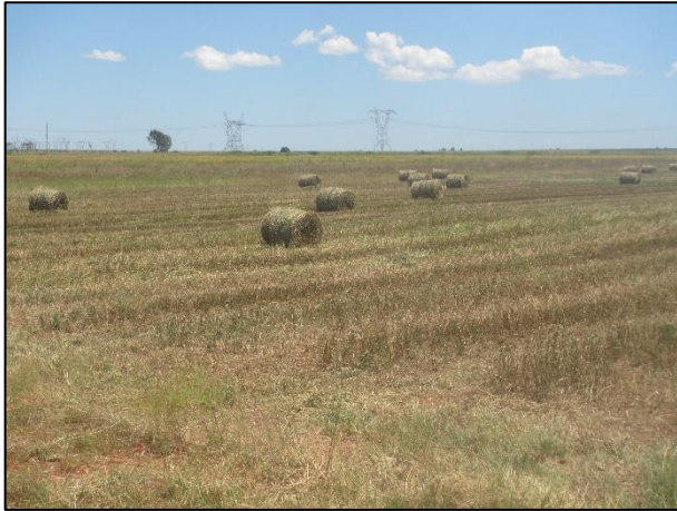
Figure 8: View across the substation site showing active fields.
