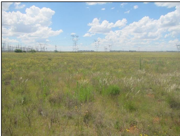
Figure 10: View north in the northern part of the powerline route with Perseus Substation visible in the background.
