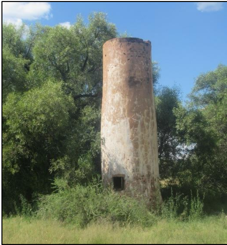
Figure 17: Ruined structure at waypoint 728.
