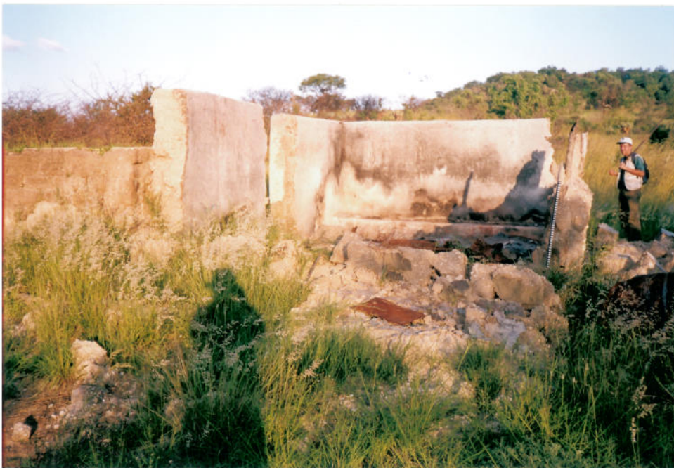
Figure 5: Site no. 5: Farm workers house showing back bench in room.
