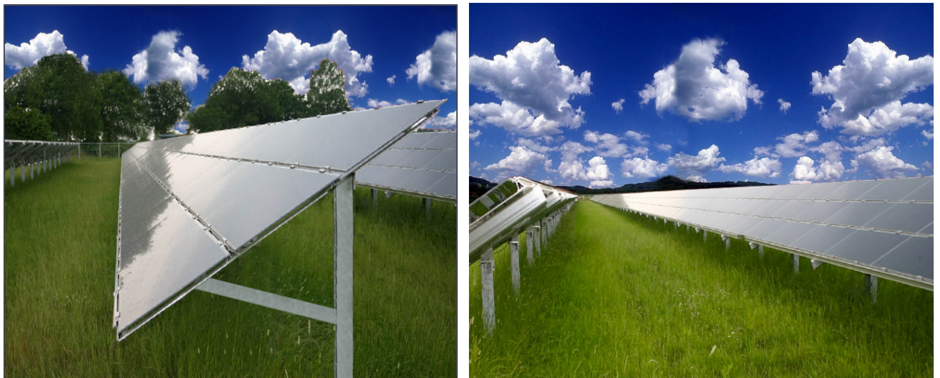
Figure 5: Lateral views of PV arrays mounted on fixed mounting systems
