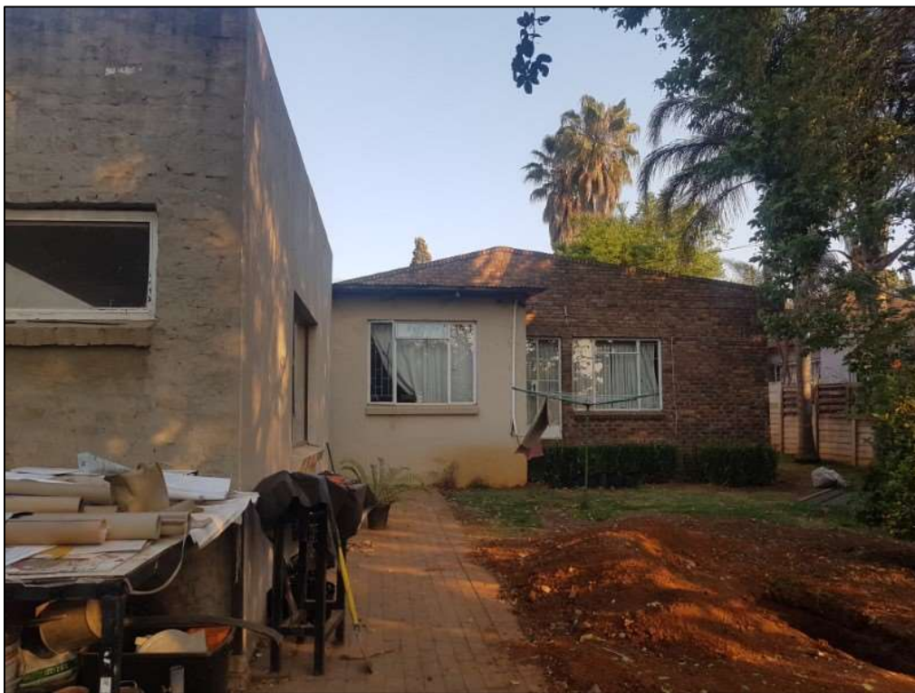
Figure 12: Erf 1/258 seen from NW to SE.
