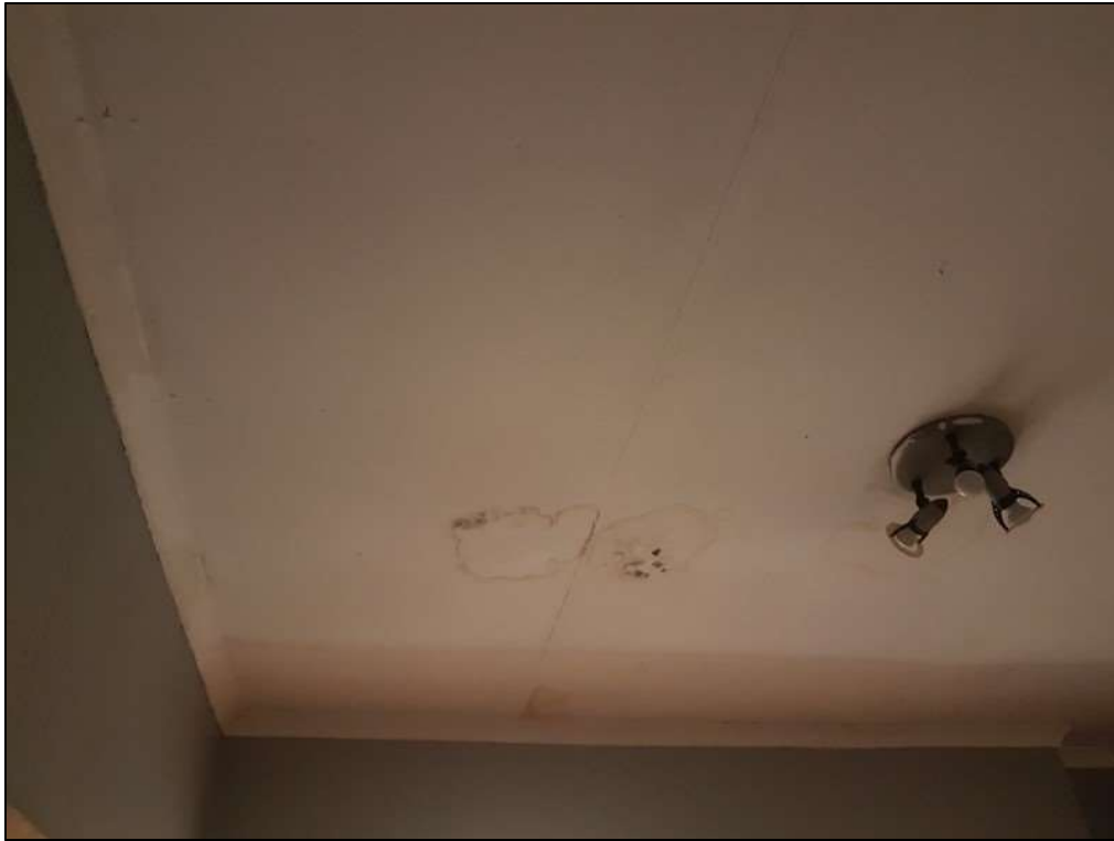
Figure 16: Water damage on the ceiling.
