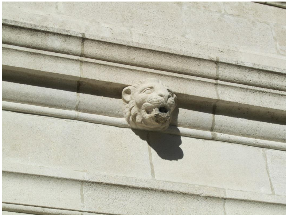
Figure 72: Gargoyle detail of the main memorial
