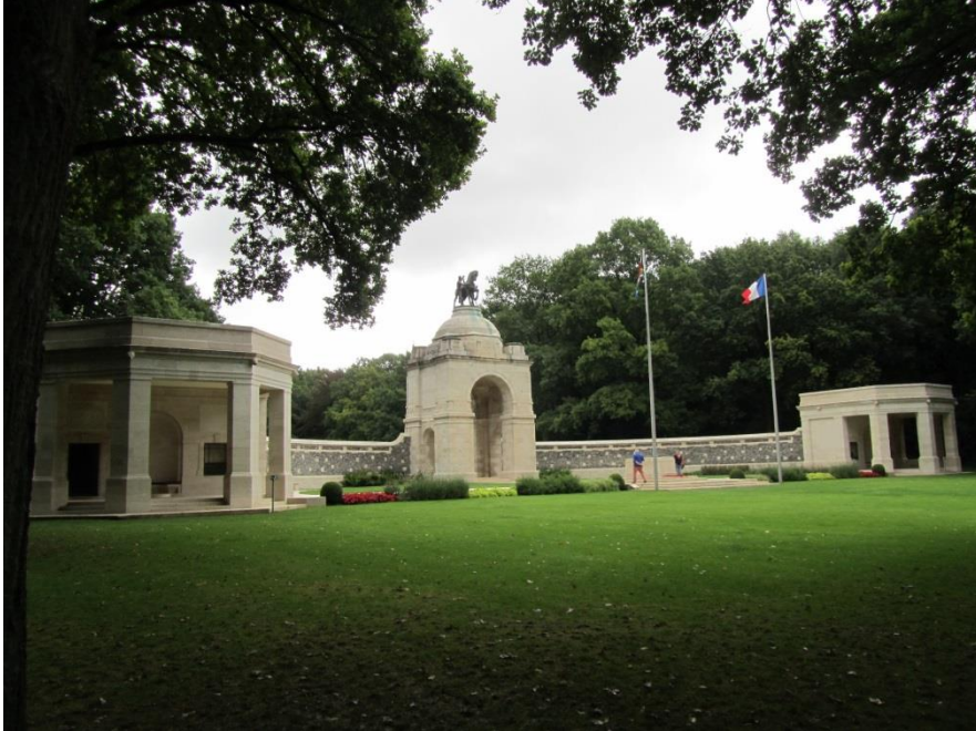
Figure 48: The southern elevation of the 1926 South African National Memorial which sits at the end of a tree lined avenue
