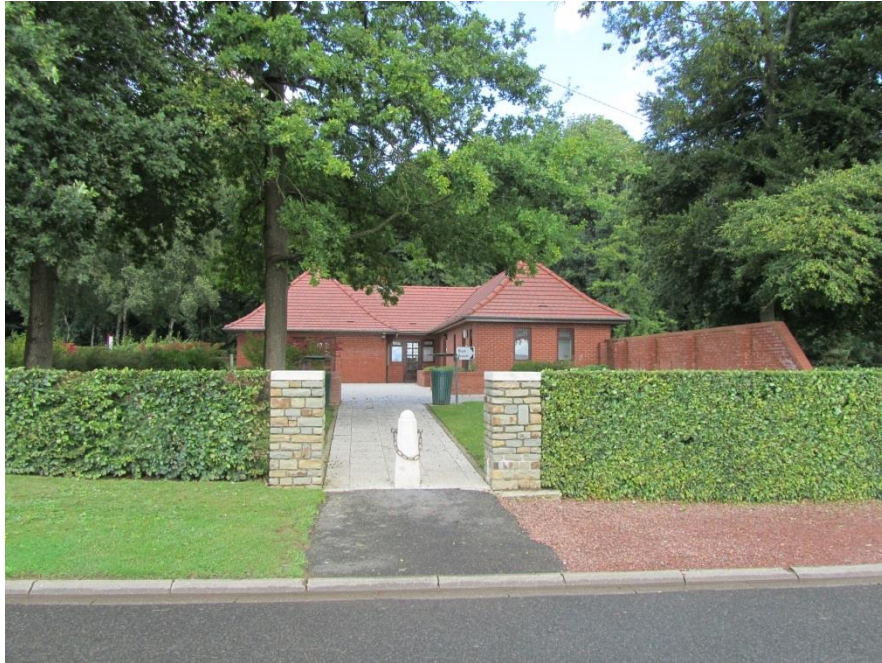
Figure 36: The Visitors Centre, circa 1984, as seen from the Ginchy Road. The care takers cottage is located to the east (right) of the visitors centre.
