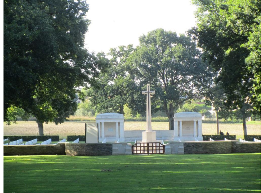
Figure 53: View down the main axis looking towards the cemetery with the cross of sacrifice and chapel shelters.
