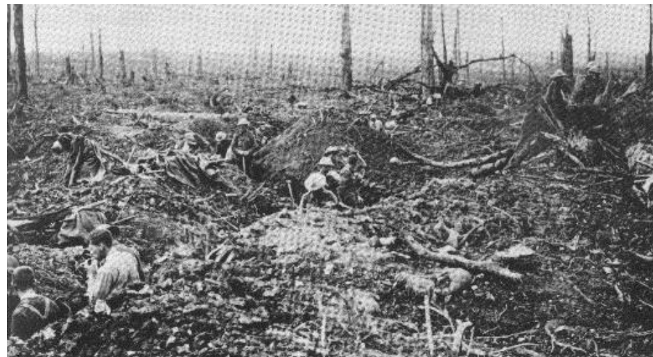
Figure 6: A communication trench being dug through the remains of Delville Wood (Uys 1983:151)
