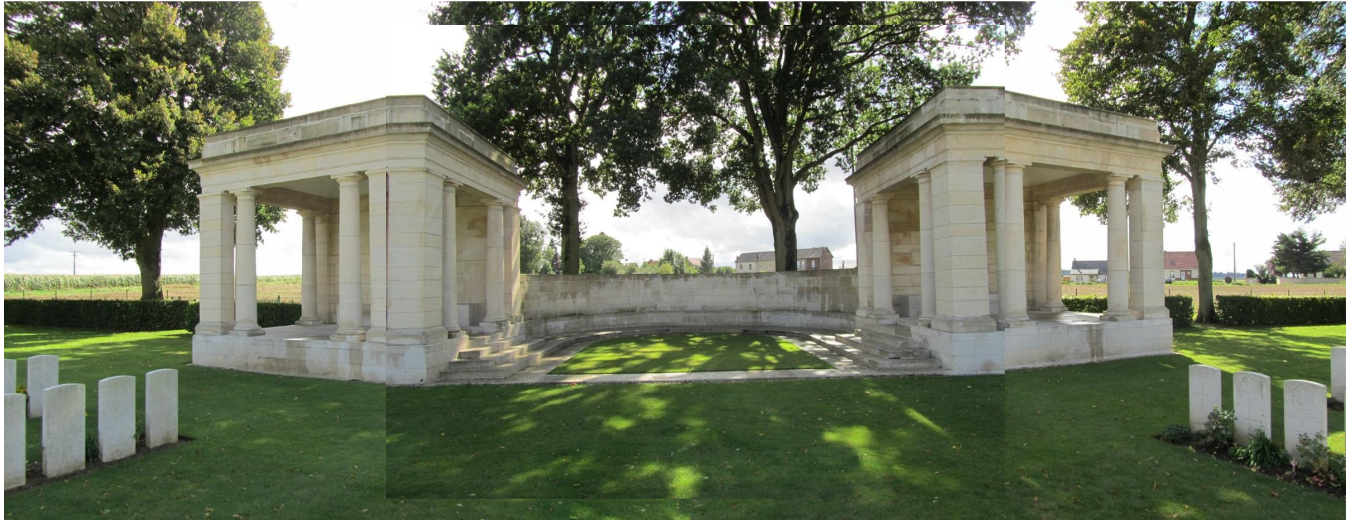
Figure 47: The two chapel shelters with the apse formed between them terminating the central axis of the cemetery
