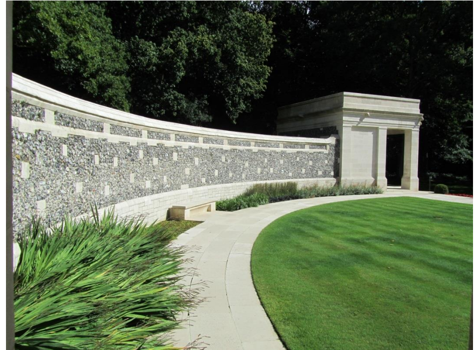
Figure 63: The semi-circular flint and sand stone wall of the memorial.
