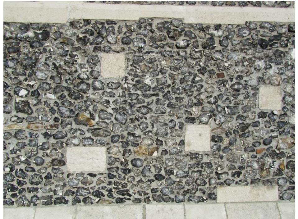
Figure 73: Detail of the flint and sand stone wall of the main memorial
