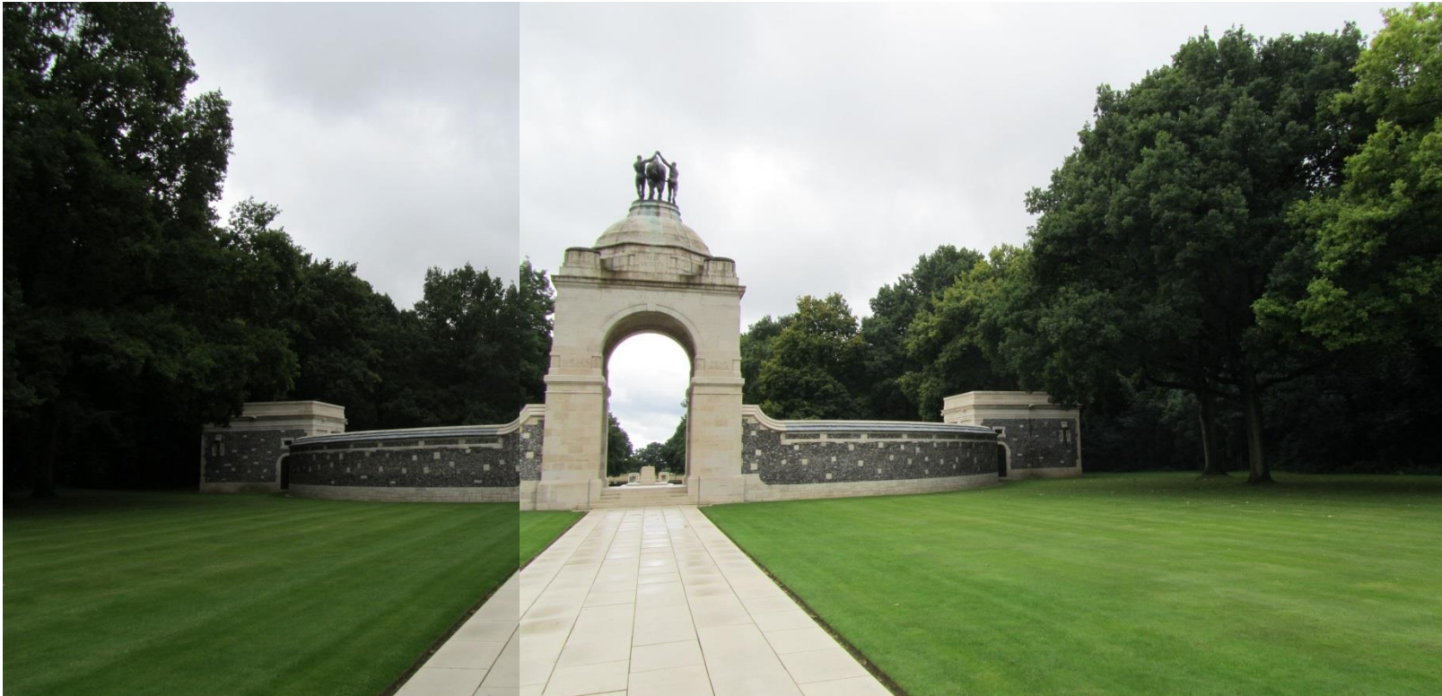
Figure 57: Composite image of the northern elevation of the arch. The image is taken from path to the museum.
