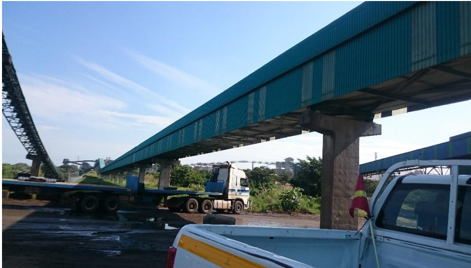
Figure 4: Left: View along the Hillside Aluminium conveyor from Transfer Tower 3 towards Transfer Tower 4. Scaffolding and/or crane will be required within the vicinity of Transfer Tower 3 (completely transformed area) to insert pipe sections into the conveyor belt. Right: View of the Hillside Aluminium conveyor belt towards Transfer Tower 3. Note the adjacent Grinrod pipe gantry.
