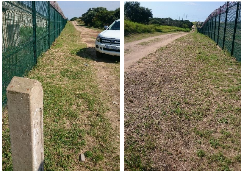
Figure 7: Once the pipeline exists to the north of the John Ross Highway, the raw water pipeline will then exist the servitude and run adjacent to the Hillside Aluminium boundary fence in a westerly direction. Left: The below ground Sasol Gas pipeline also runs adjacent to the Hillside Aluminium fence line. Right: View back towards the culvert under the John Ross Highway along the Hillside Aluminium southern boundary fence line.
