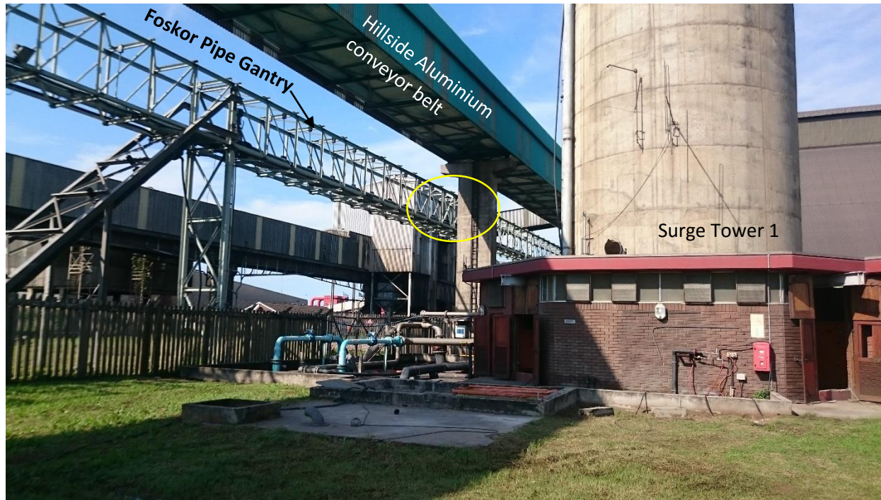
Figure 3: The Foskor pipe gantry runs parallel to the Hillside Aluminium conveyor belt. The Tee off (shown in yellow) will be created (at Surge Tower 1) for the dedicated Hillside Aluminium raw water pipeline feed to continue within the Hillside Aluminium conveyor system to the smelter. The pipe will be connected to the back (south side) of the concrete support strut. Scaffolding and/or crane/ cherry picker will only be utilised within this area (the Surge Tower 1 footprint – highly disturbed area). Pipes will be “pulled” and “pushed” within the conveyor and joined together within the conveyor to remove all external works/ scaffolding required.
