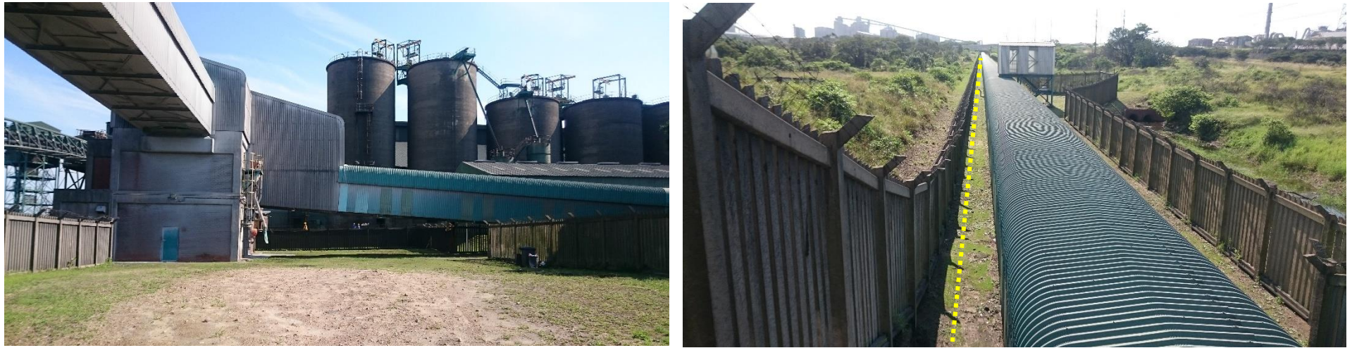
Figure 6: Left: Transfer Tower 4. Here the pipeline will exit the conveyor belt and be laid aboveground to the left of the conveyor belt running in a north-easterly direction to the Hillside Aluminium smelter. Right: The entire conveyor belt is contained within a fenced servitude. The raw water pipeline will be laid aboveground to the left of the conveyor (as indicated in yellow).
