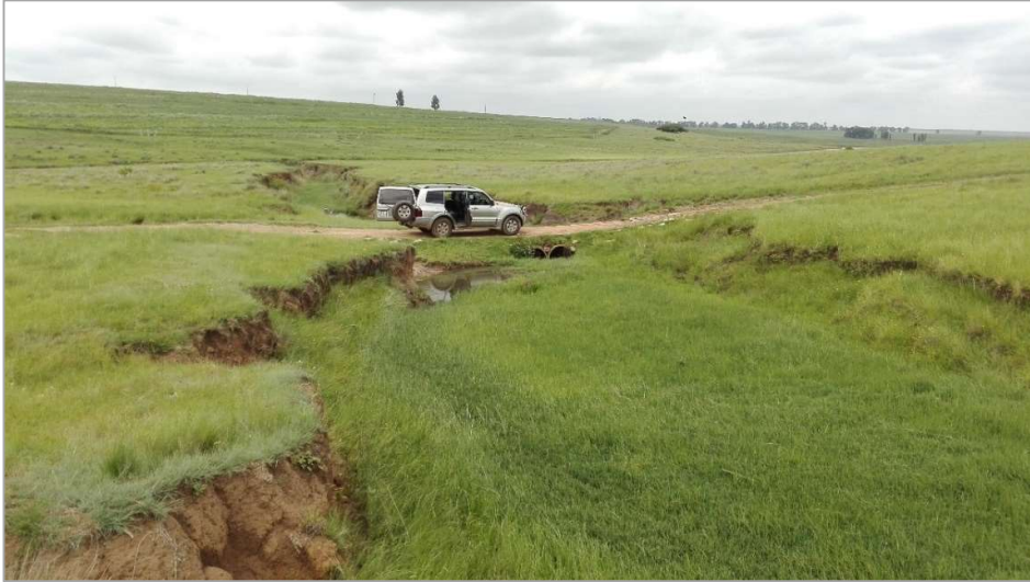
Figure 26: Photo of existing access road crossing Hillslope Seep (Alternative 1)
