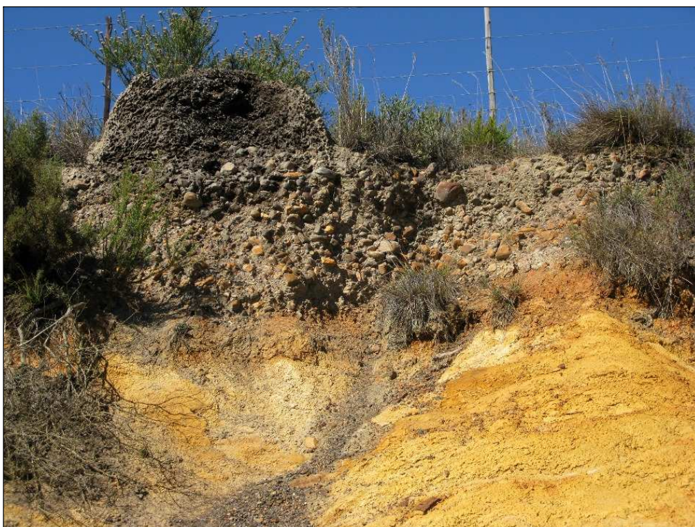
Fig. 19. Pebbly soils overlying weathered Bokkeveld Group saprolite, R62 road cutting (Loc. 048). The high degree of pebble rounding suggests fluvial transport.
