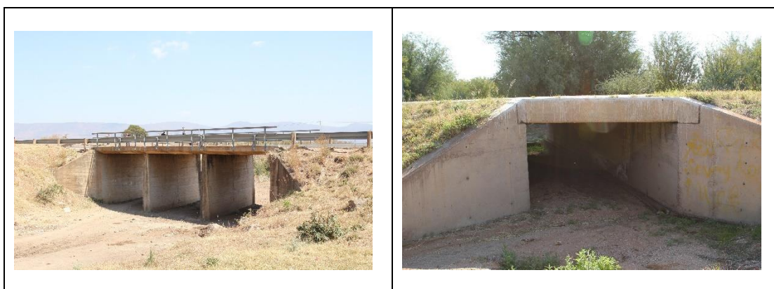
Figure 9. Examples of bridges of similar material and construction
