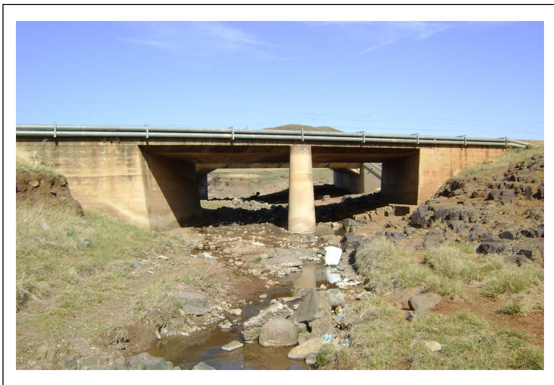
Figure 1. Side view of the Mbokotwana River Bridge (Eastern aspect)
