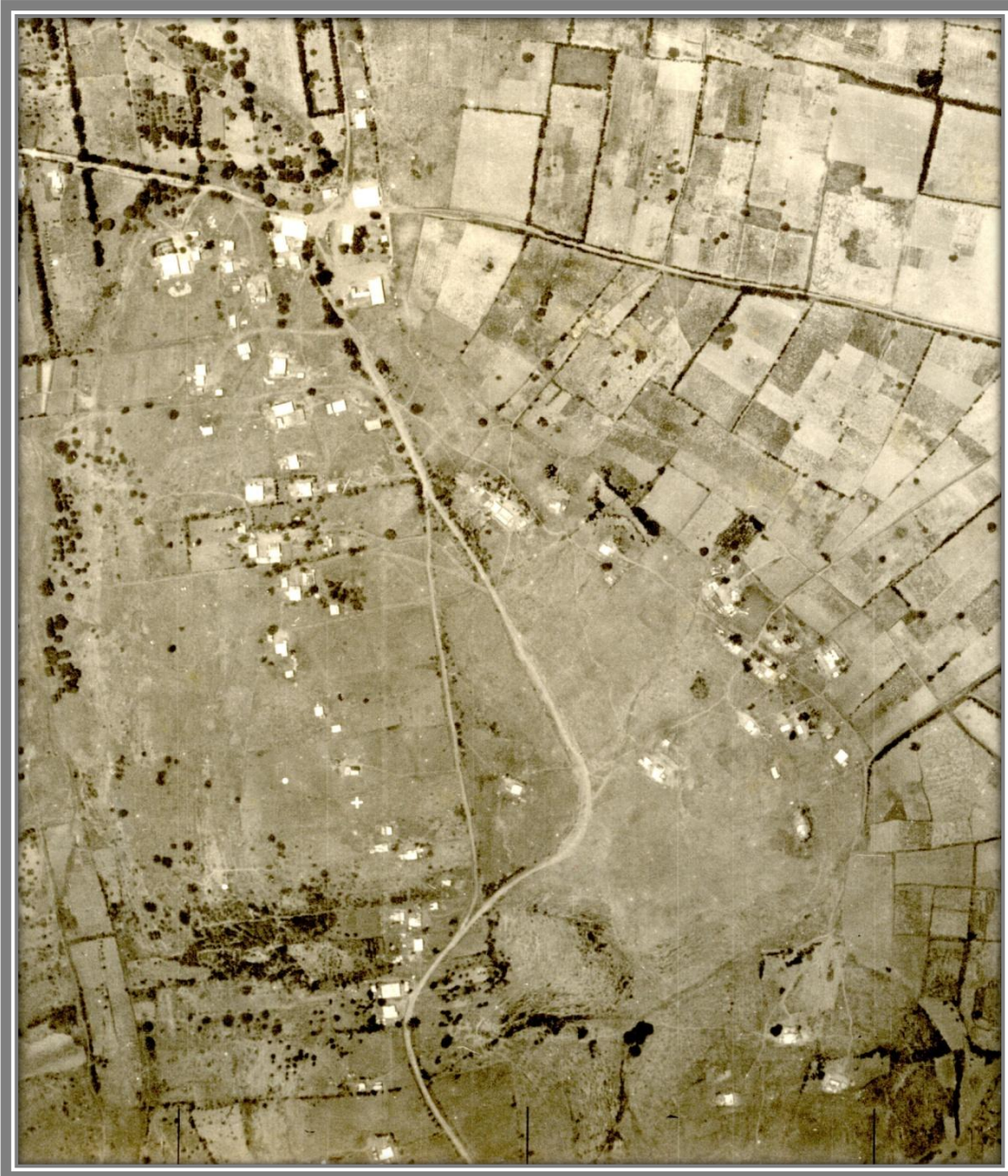
FIGURE 5 AERIAL PHOTOGRAPH OF DEVELOPMENT SITE IN 1931.
