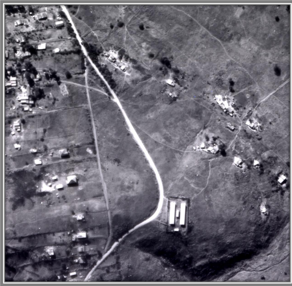
FIGURE 6 AERIAL PHOTOGRAPH OF DEVELOPMENT SITE IN 1949.
