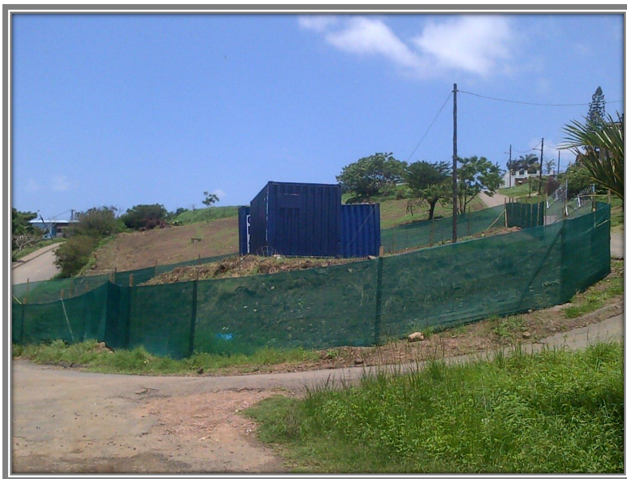
FIGURE 11 EARTHWORKS ON SITE IN DECEMBER 2013 (SOURCE: AMAFA).
