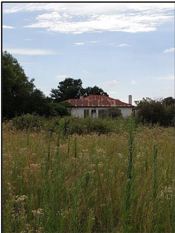
Figure 9.23. West facing wall of the original farmhouse.
