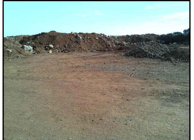
Figure 10: Earth works at the existing quarry.
