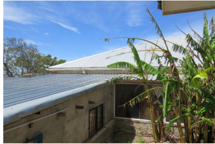
Roof of unit from courtyard
