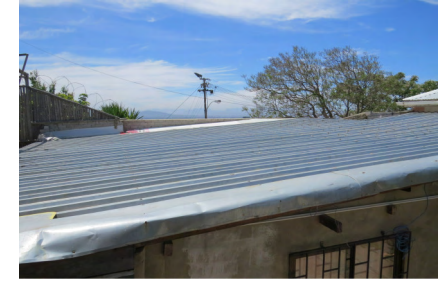
Roof of unit from courtyard
