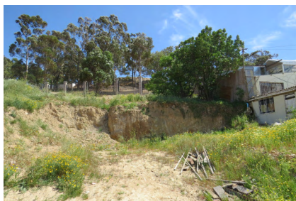
Unfinished earth works
