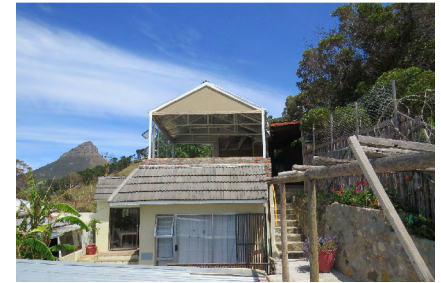
Framed structure above unit
