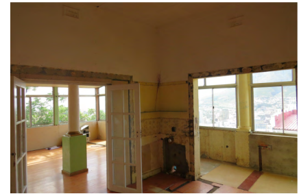
Double doors to living room
