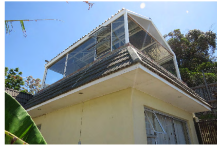
Framed structure above unit
