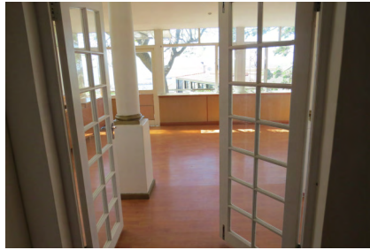
Double doors to living room
