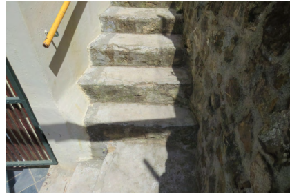
Steps along boundary wall
