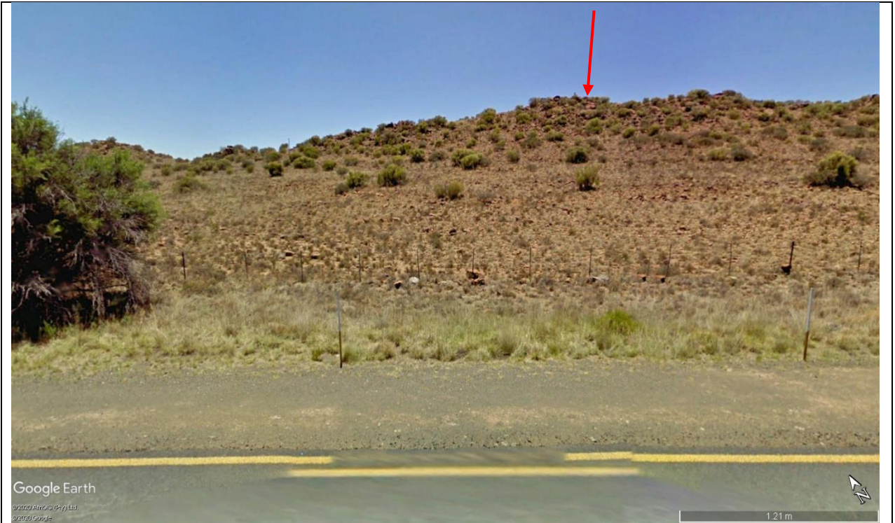
Figure 2: Google Earth Street View from the N10 showing the approximate location of the telecommunications mast.
