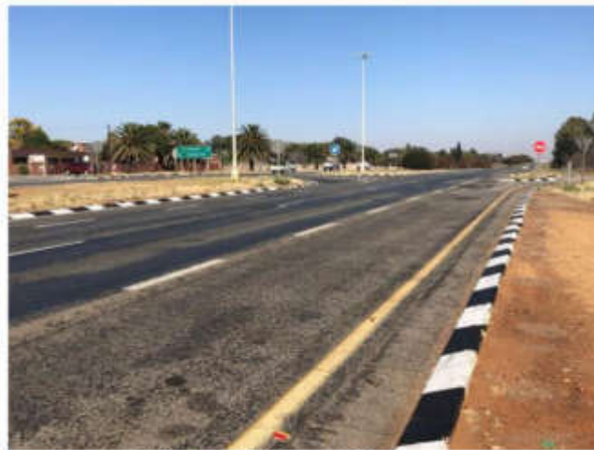
High mast lighting on N12
