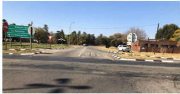
Intersection N12 and Kowie Street direction South
