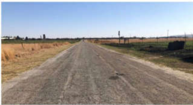
Kowie Street with the site on the right
