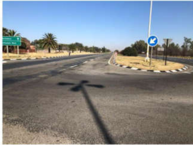
Axillary lane on N12 to be widened
