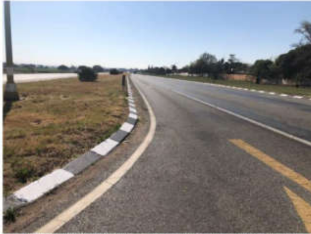
Right-turn lane on N12 eastern approach to be widened
