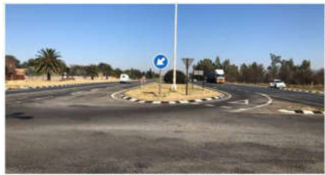
Intersection N12 and Kowie Street direction East
