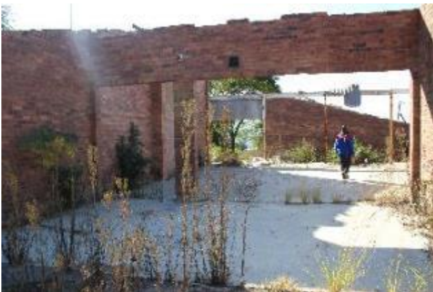
Figure 15: Interior of Site Complex 2.
