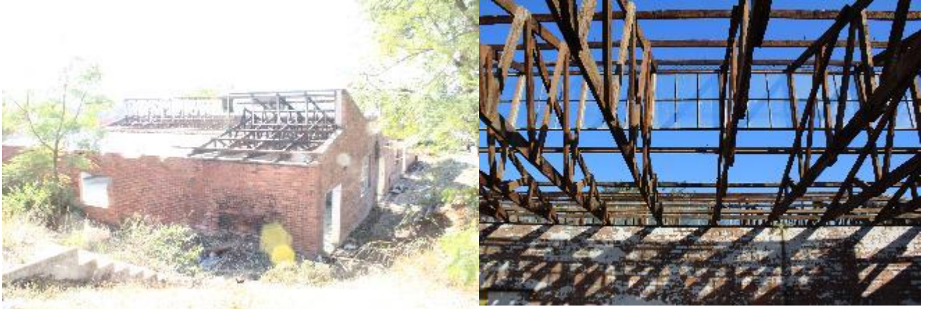
Figure 18: Roof stripped of buildings in Site Complex 3.
