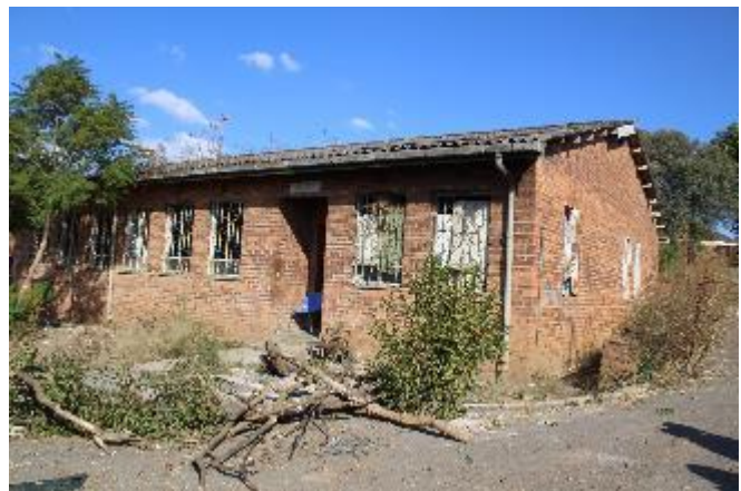
Figure 20: Exterior of one of the buildings in Site Complex 4.
