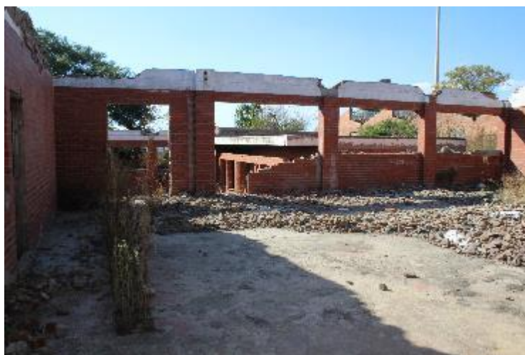
Figure 13: Interior of Site Complex 1
