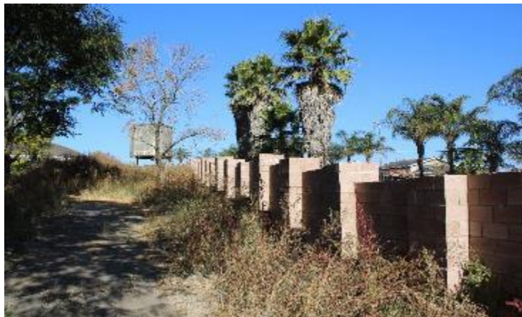
Figure 1: Photo of boundary wall.
