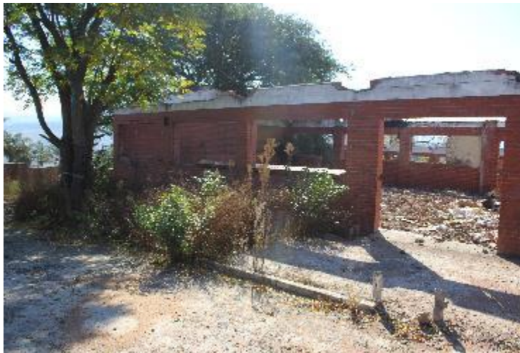
Figure 12: Site Complex 1 facing north.
