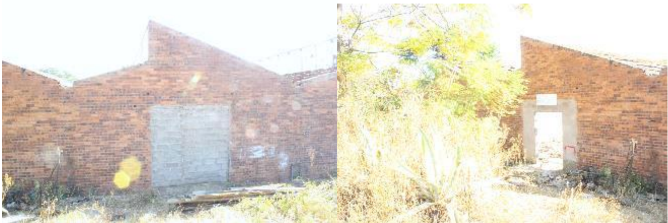
Figure 17: Exterior of Site Complex 3.
