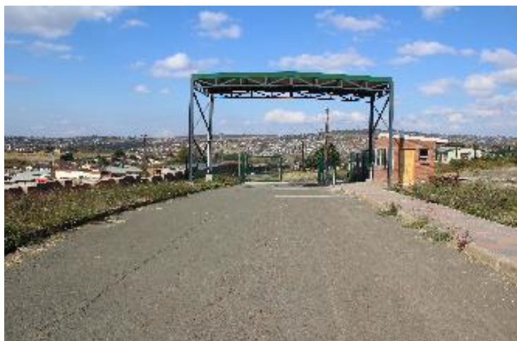
Figure 2: New security gate at the entrance of the property.
