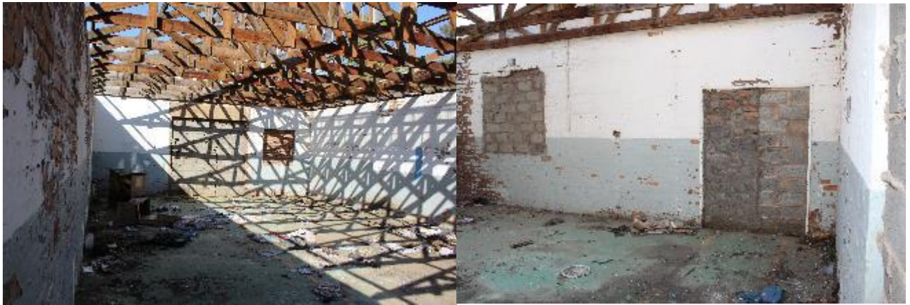
Figure 19: Interior of Site Complex 3.
