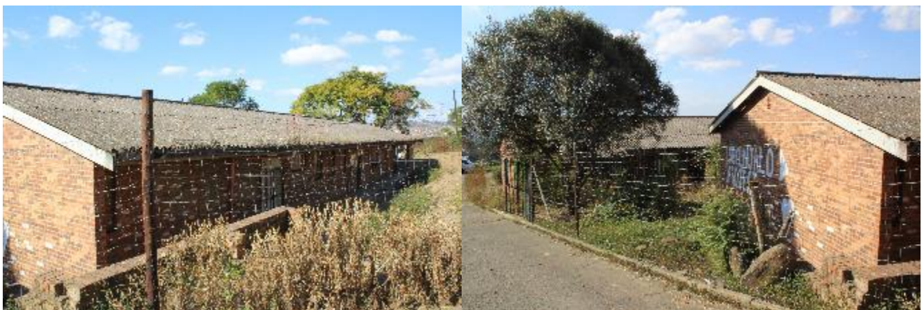
Figure 24: Buildings currently being used by the Sekunjalo Project, in Site Complex 4.
