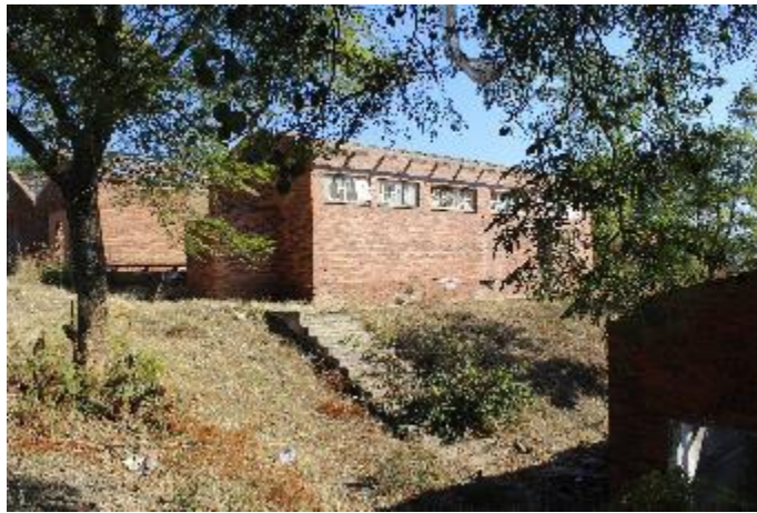
Figure 22: Another building in Site Complex 4.
