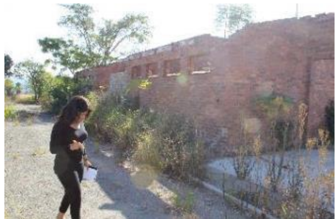
Figure 16: Exterior of Site Complex 2.
