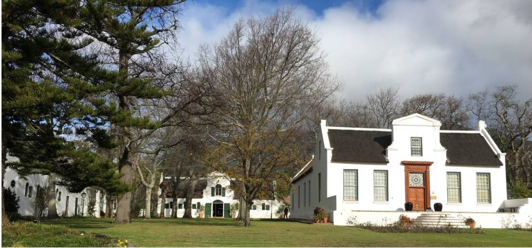
Figure 21: The north eastern side of the U-shape complex. The complex turns its back on the site of the dam. The former wine cellar is the closest building with its main facade facing north east
