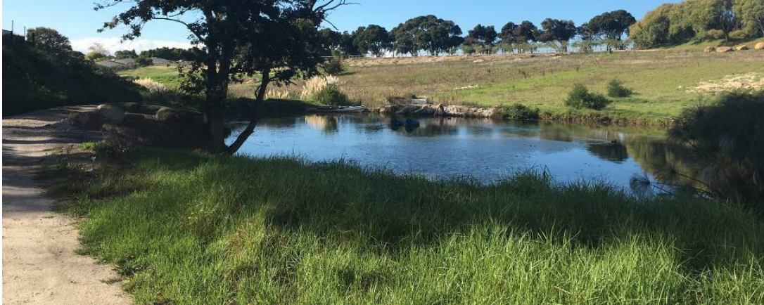
Figure 14: The main dam which was probably constructed before 1966
