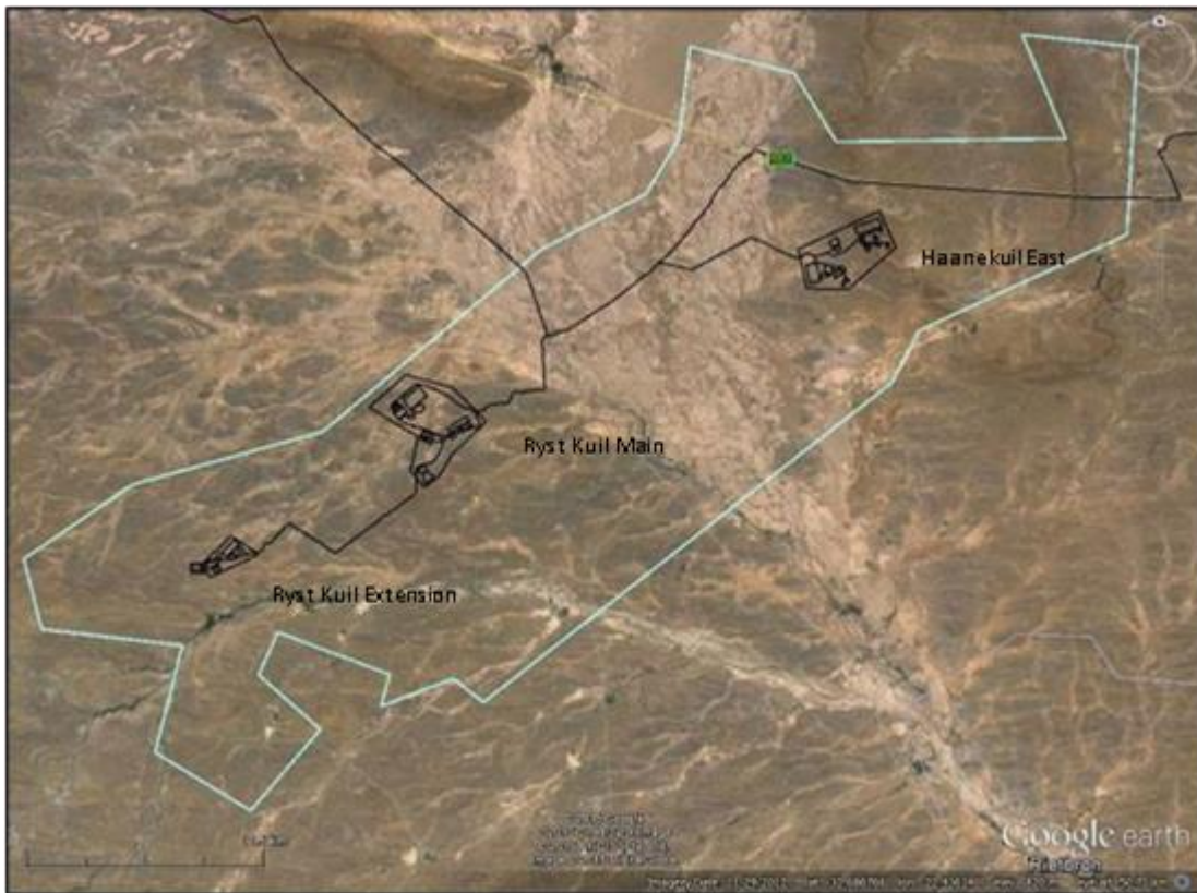
Figure 5: The extent of mining and mining related infrastructure on Ryst Kuil (Eastern Block) to the south of the R61. It is 55 km in length and 14 km width. However, mining will only occur within three locations in this area, namely at Haanekuil East, Ryst Kuil Main and Ryst Kuil Extension.
