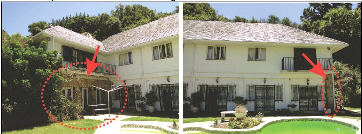
Images 1 & 2: Sections of stonewalling remaining, fenestration (to left) suggests original structure was single storey height
