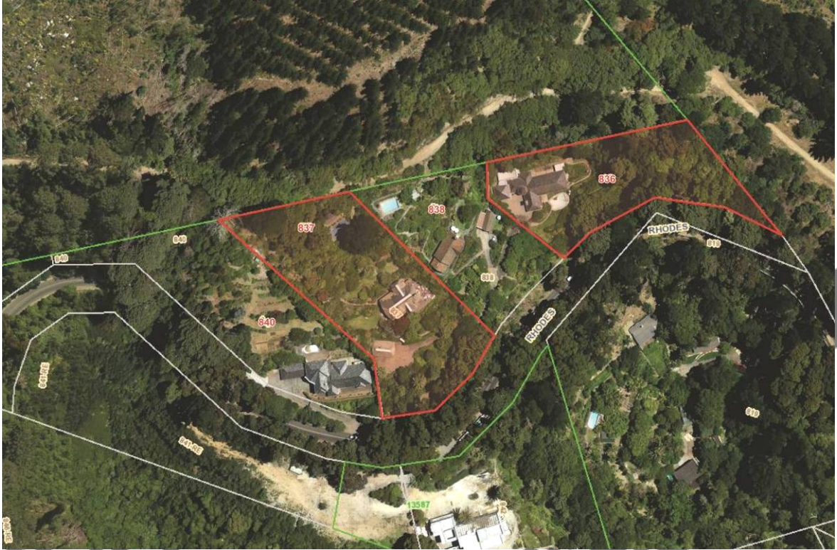
Figure 2: Contextual aerial image of Erven 836, 837 illustrating sylvan setting. Note modern residence here visible on Erf 840, which had been demolished during 2013 (Source: CoCT, 2012)
