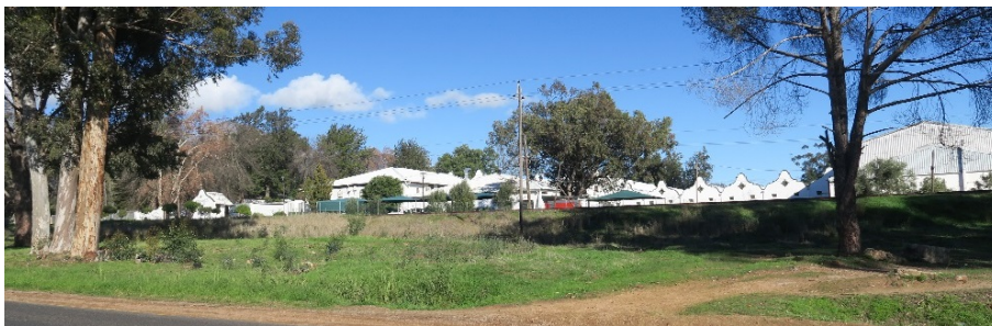
Figure 46: From the R45 the gabled warehouses are however largely screened by the ('intrusive and negative') buildings situated in the foreground and the elevated railway line.
