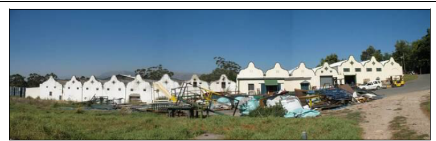
Photograph 2.16a: Historic Barns, western (rear) elevation, 2008 ACO
