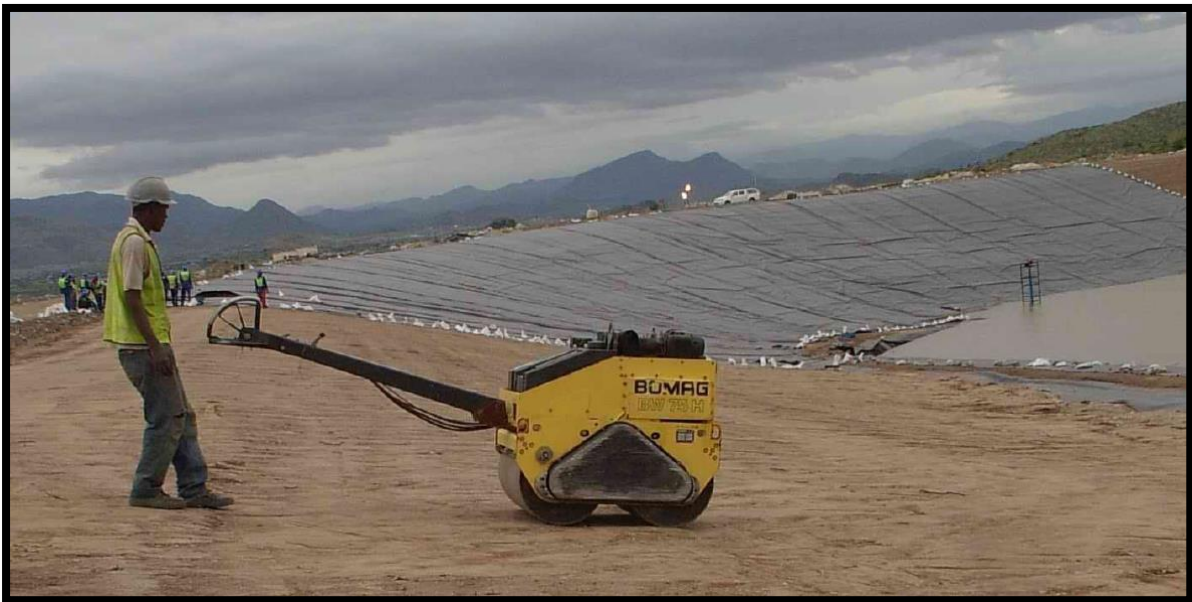
Figure 3-5: Construction taking place on the TDF
