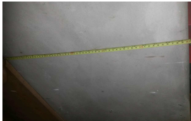
Photo 4.3.3 & 4.3.4: Downstand Reinforced Concrete Ring beam inside basement ( 700dp x 600 wide)
