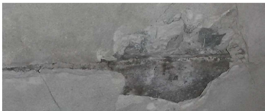
Photo 4.4.3: Exposed steel beam with almost no visible corrosion
