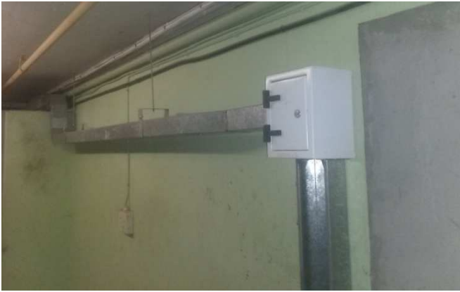
Photo 4.6.22: Passage 2 - More services inside basement
