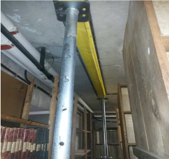
Photo 4.2.1: Existing props and spreader beams in basement
