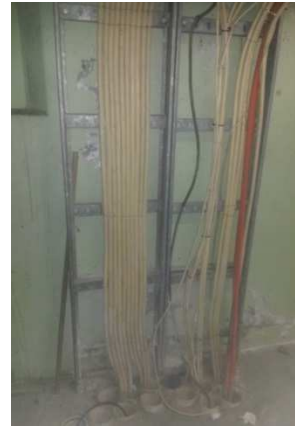
Photo 4.6.23: Passage 2 - Numerous Service sleeves in the basement floor
