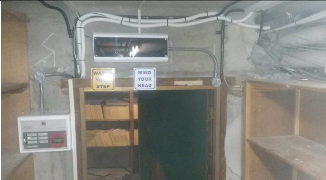
Photo 4.6.16: Passage 3 – Basement timber door
