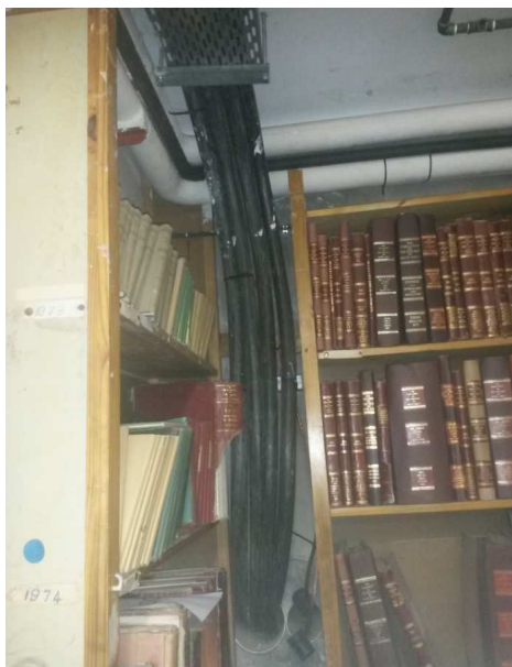
Photo 4.5.36 & 37: 4x Black PVC conduits entering the basement on the near left corner of the basement
