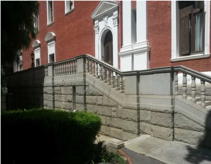
Photo 4.6.1: Granite cladded wall at side entrance staircase to external balcony
