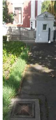
Photo 4.6.14: Storm water manhole close to basement
