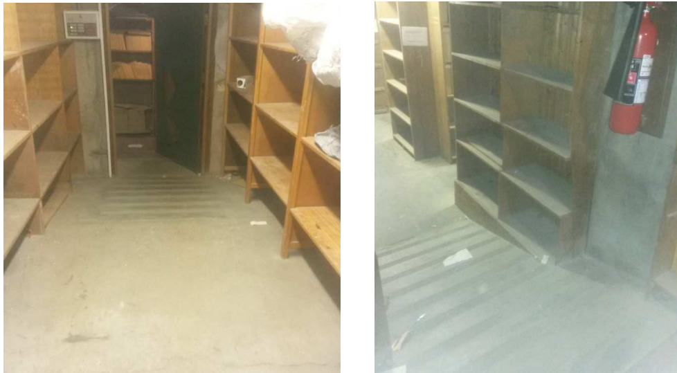
Photo 4.6.17 & 18: Passage 3 – Basement entrance door with ramps down either sides of doorway
