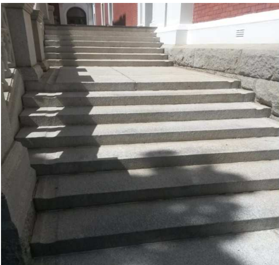
Photo 4.6.3: Granite cladded steps with grooves either sides for rainwater run-off
