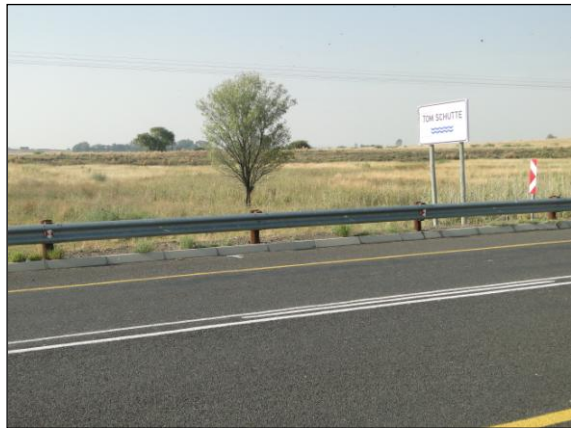
Plate 6: Dam wall in the background on the eastern side
