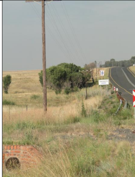
Plate 2: Closer view towards Tom Schutte Bridge
