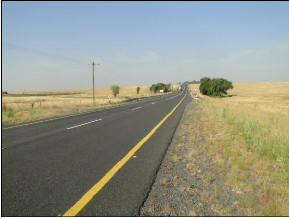
Plate 1: View towards Tom Schutte Bridge
