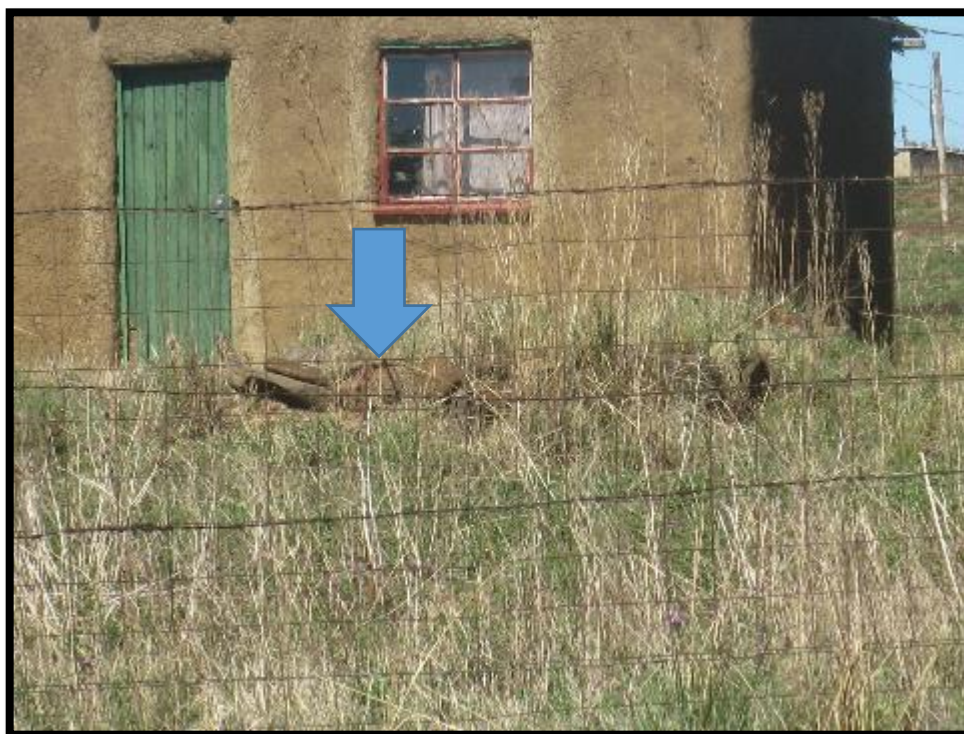
Figure 12. Grave Site 2: situated directly adjacent to an occupied residential dwelling.
