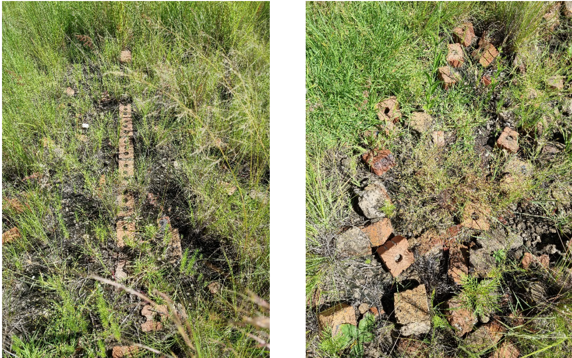
Figure 20: Building from UP-DRF-2529-02.
