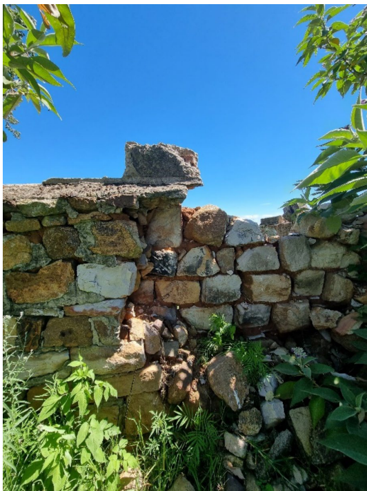
Figure 15: UP-2529-DRF-01 indicating (a) broken rubble fill wall in space 3 and (b) daga plaster and fill.
