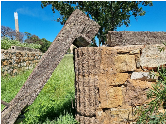
Figure 17: UP-2529-DRF-01 with (a) doorway into Area 3 showing with corrugated imprints in cement and (b) building rubble and corrugated asbestos roofing sheet north of the UP-2529-DRF-01.
