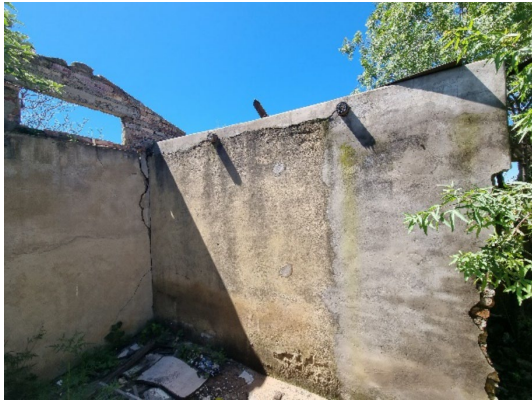
Figure 13: Area 1 of UP-2529-DRF-01 facing (a) towards the south east with gum pole visible in interior room wall and (b) facing towards the north with impressions left by gum poles on cement wall cap.
