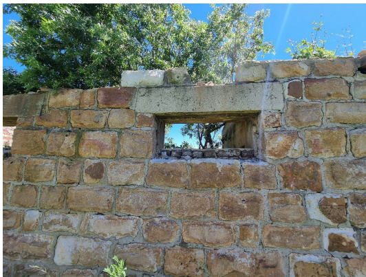
Figure 14: UP-2529-DRF-01 ith view of corase sandstone walls; (a) outside, facing north with cement lintel and (b) standing in Area 2, facing south showing northern wall of Area 1.
