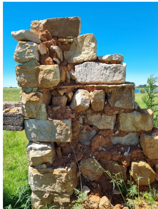
Figure 15: UP-2529-DRF-01 indicating (a) broken rubble fill wall in space 3 and (b) daga plaster and fill.
