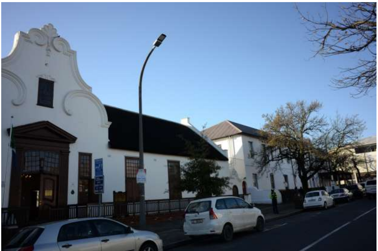
Street context: Looking north-east along Alexander Street (the 1930's Cape Dutch Revival Cape Winelands District Municipality building is on the left)
