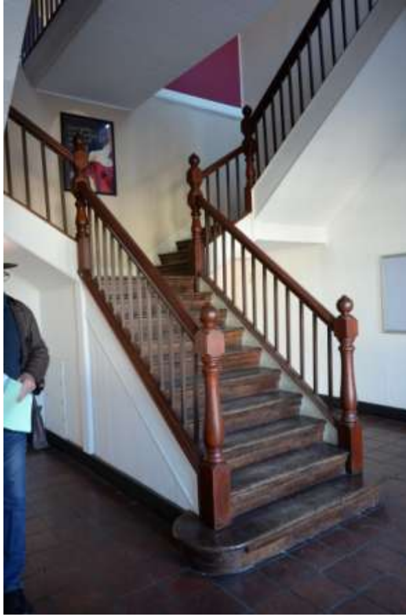
The timber staircase
