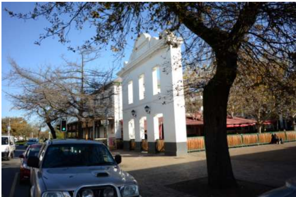
The Heuer building façade on Bird Street
