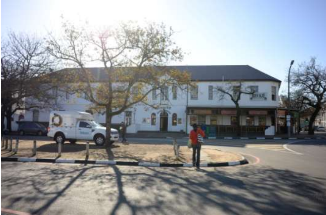
View from Alexander Street looking north
