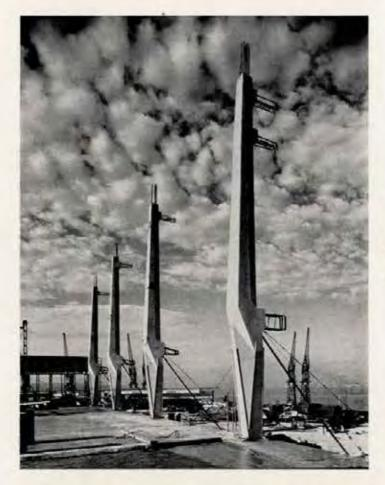
Carefully designed precast concrete columns being erected to support the main concourse.
