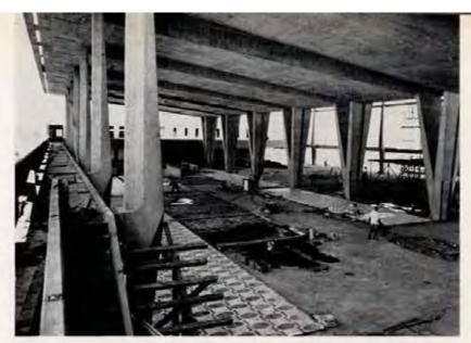
Main concourse under con-struction showing precast columns in position and terrazzo floor slabs being laid.
