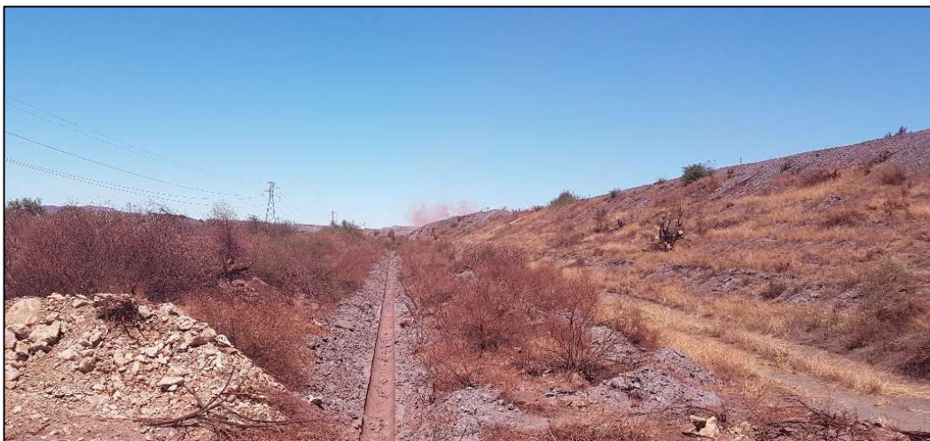
Figure 5: Existing asbestos-lined solution trench at the toe of the tailings dams
