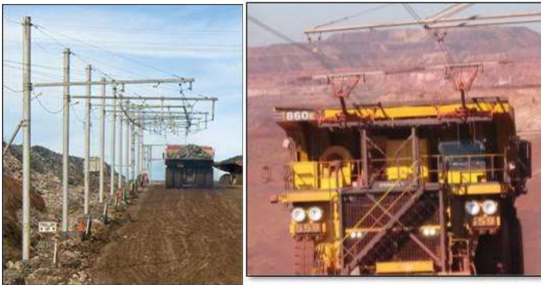
Figure 9: Trolley assist infrastructure
