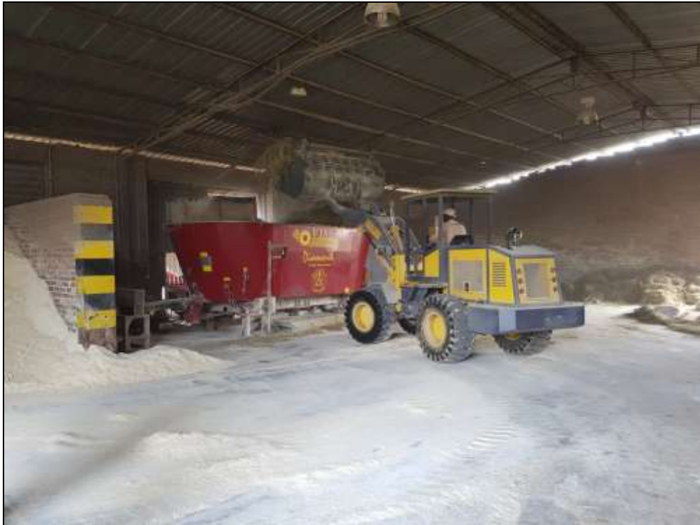
Fig. 3. General site conditions. Plant and equipment on the abattoir site
