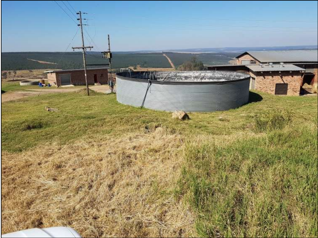
Fig. 5. General site conditions. Existing facilities and buildings.
