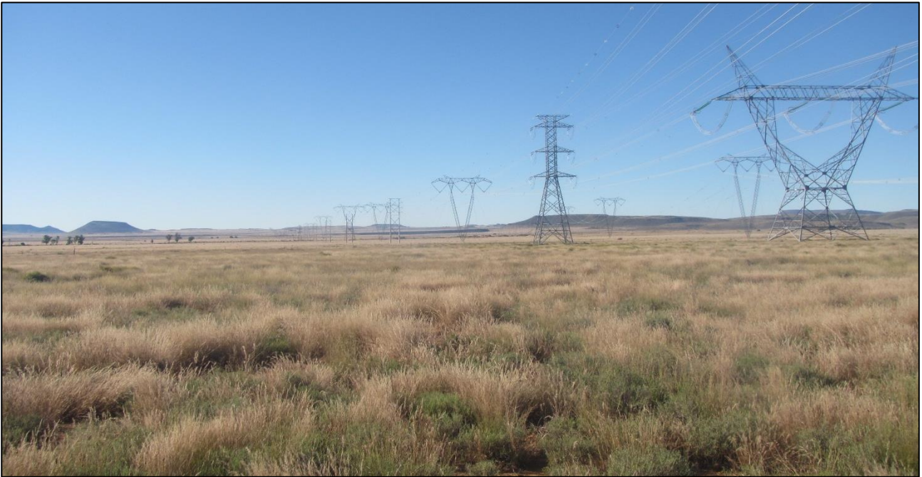
Figure 7: View towards the northeast along the north-eastern part of the PV1 Alt. 1 corridor. This view looks from the farm fence across the land that was not accessible for the survey.
