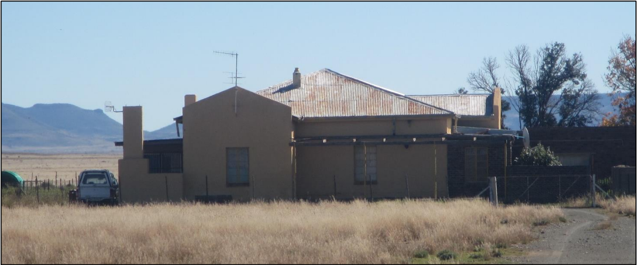
Figure 28: Farmhouse at waypoint 932.
