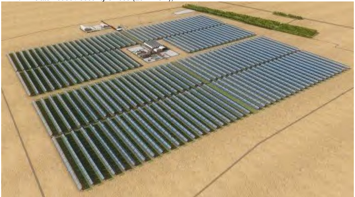
Figure 3: Typical layout of the components of a Solar PV facility (Source: Cape_EAPrac, October 2014)
