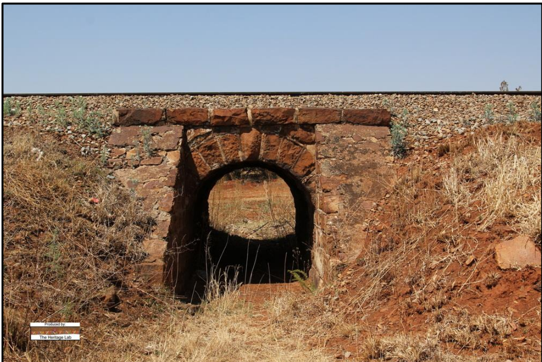
Figure 7. Stone railway culvert on the Potchefstroom line (1897), located west of the project area
