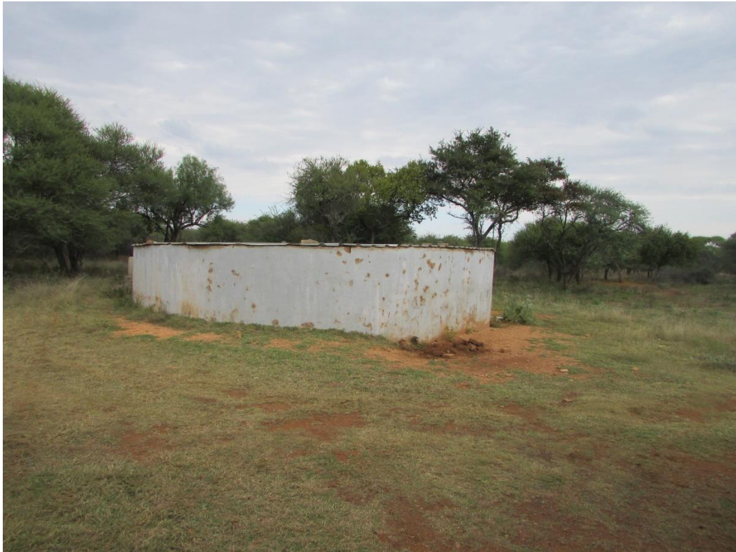
Figure 11: The Water Reservoir/dam at Site 2.
