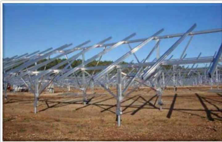
Photograph of example of mounting (Source: VRMA)
