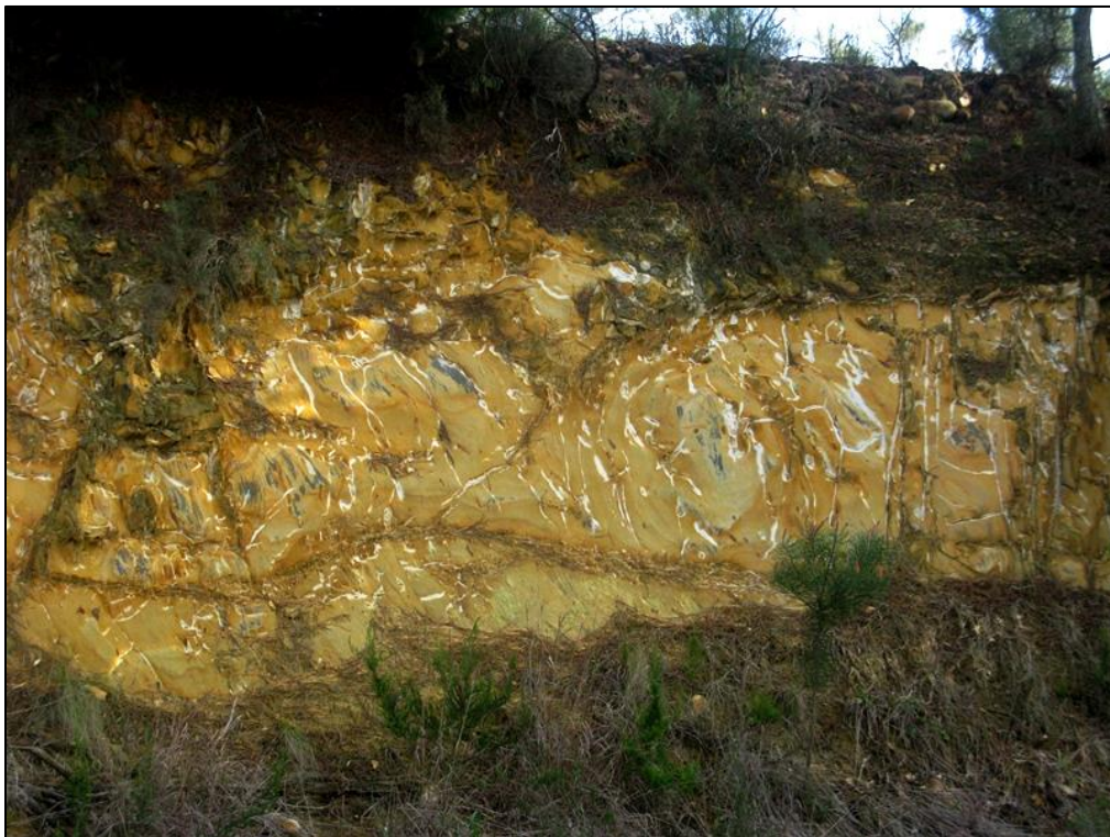
Figure 15. Deeply-weathered, mottled mudrocks of the Gydo Formation (Bokkeveld Group), R102 road cutting just west of Impofu Dam (Impofu North Wind Farm study area).
