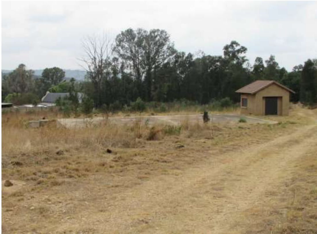
Figure 6: The line will link up with an existing sewer plant in The Hills property.
