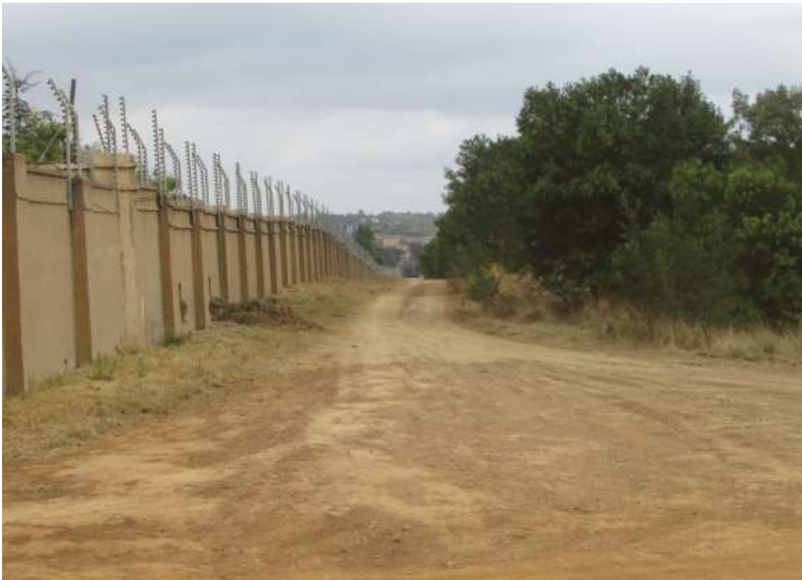
Figure 5: A section of the sewer line follows a road servitude down the boundary fence of The Hills Eco Golf Estate.
