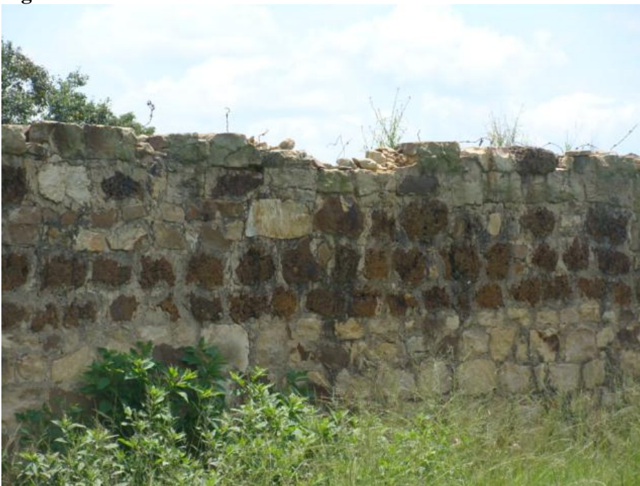
Figure 11 Close-up of one of the walls of the house.
