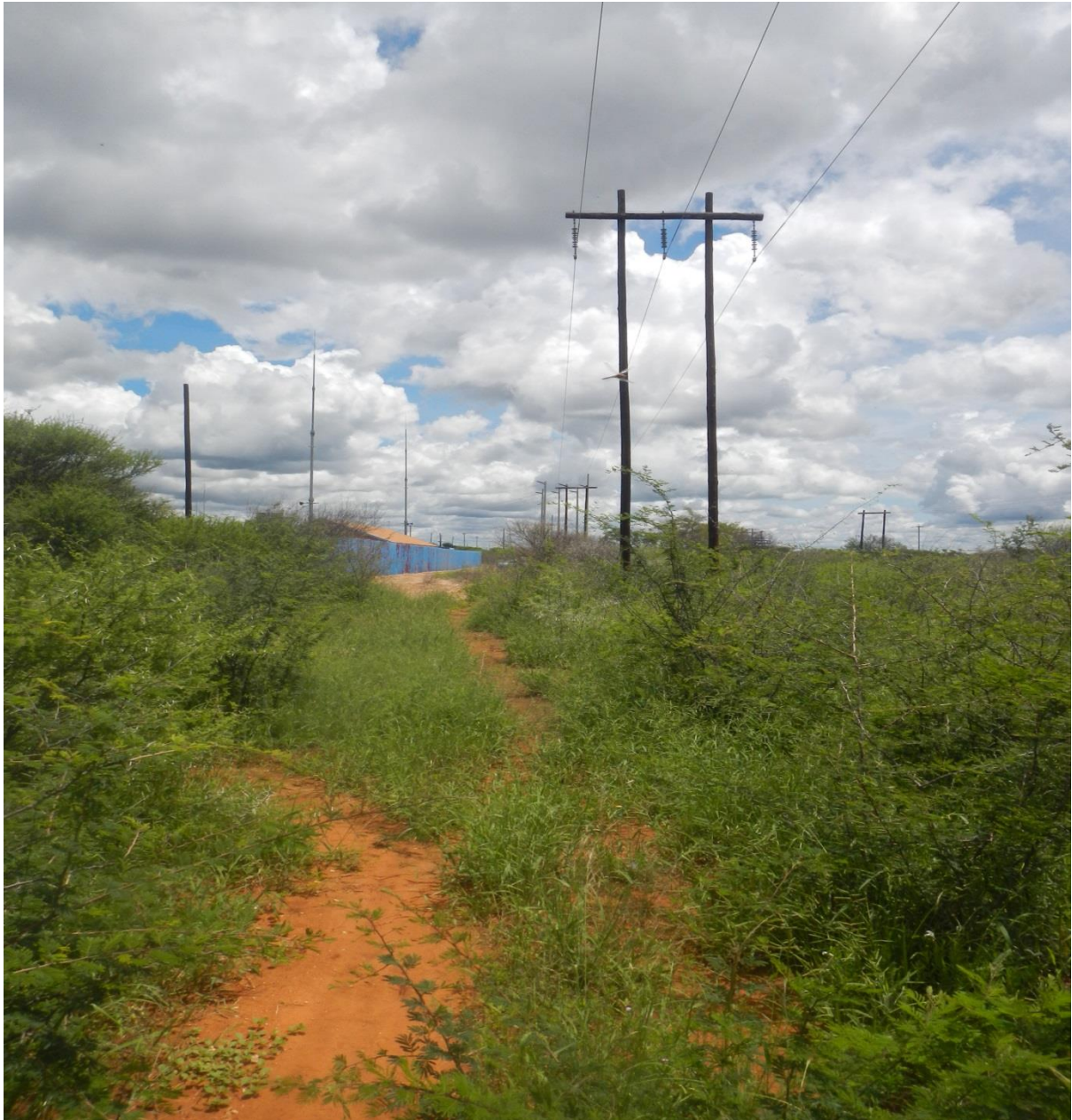
Figure 6: A view of the existing powerline with access roads
