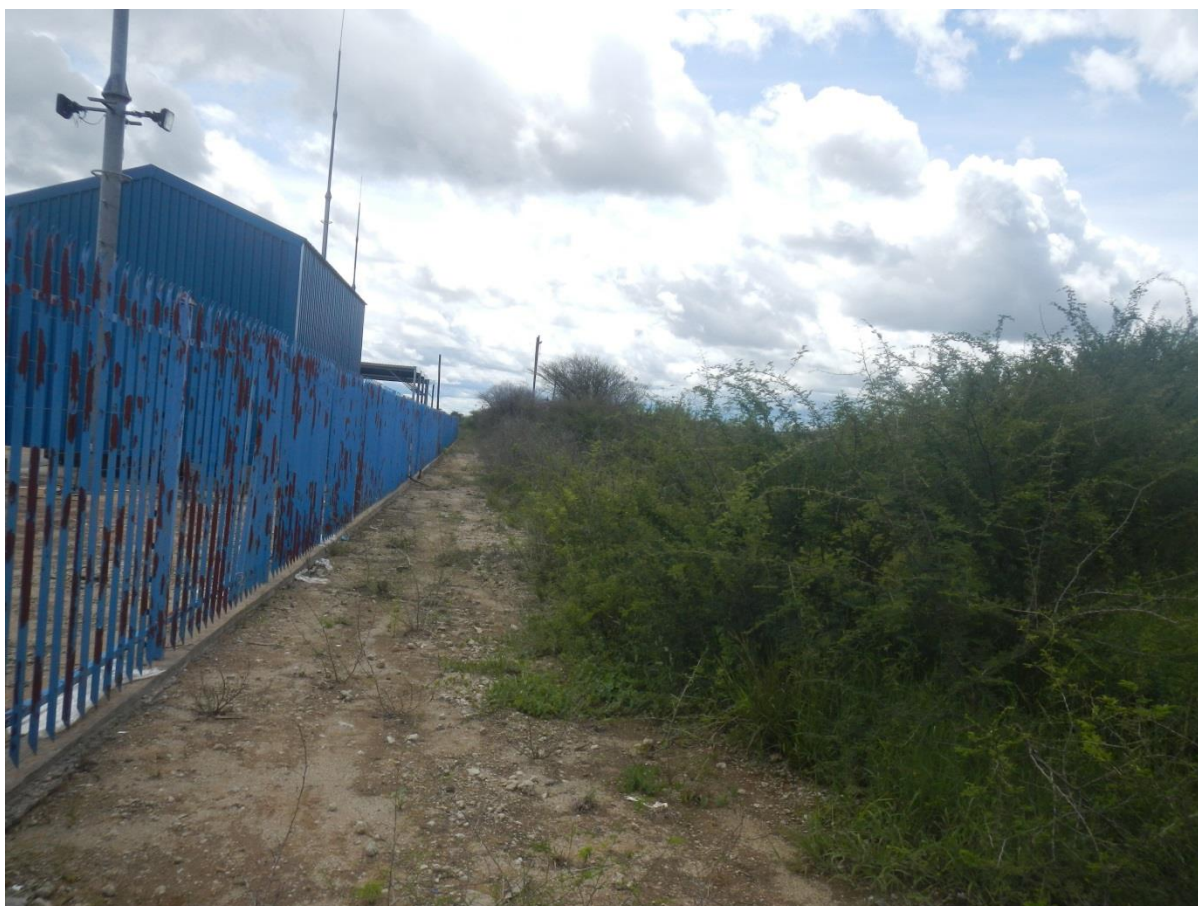
Figure 9: View of the proposed development footprint in relation to the existing substation features
