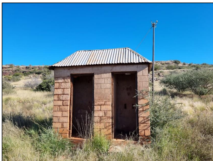
Figure 6-20: View of the small telephone booth building at NH-MG-2822-04.
