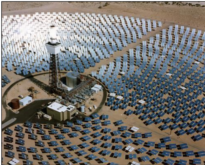
Figure 3 - An example of a power plant using central receiver technology. This is a 10MW demonstration plant that was built in the United States – image courtesy NREL.
