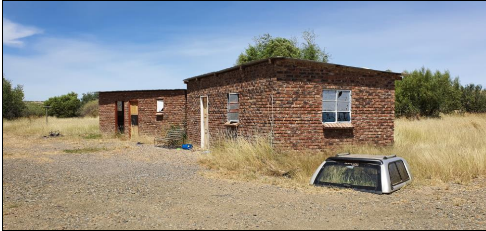
Figure 16: General view of the north section (existing infrastructure) of the survey footprint
