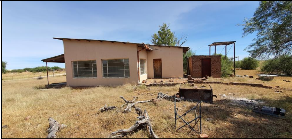
Figure 41: The eastern facade of the building
