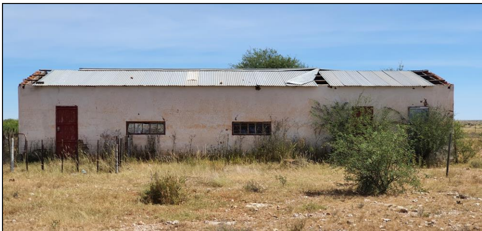
Figure 42: An outbuilding (shed) probably added later
